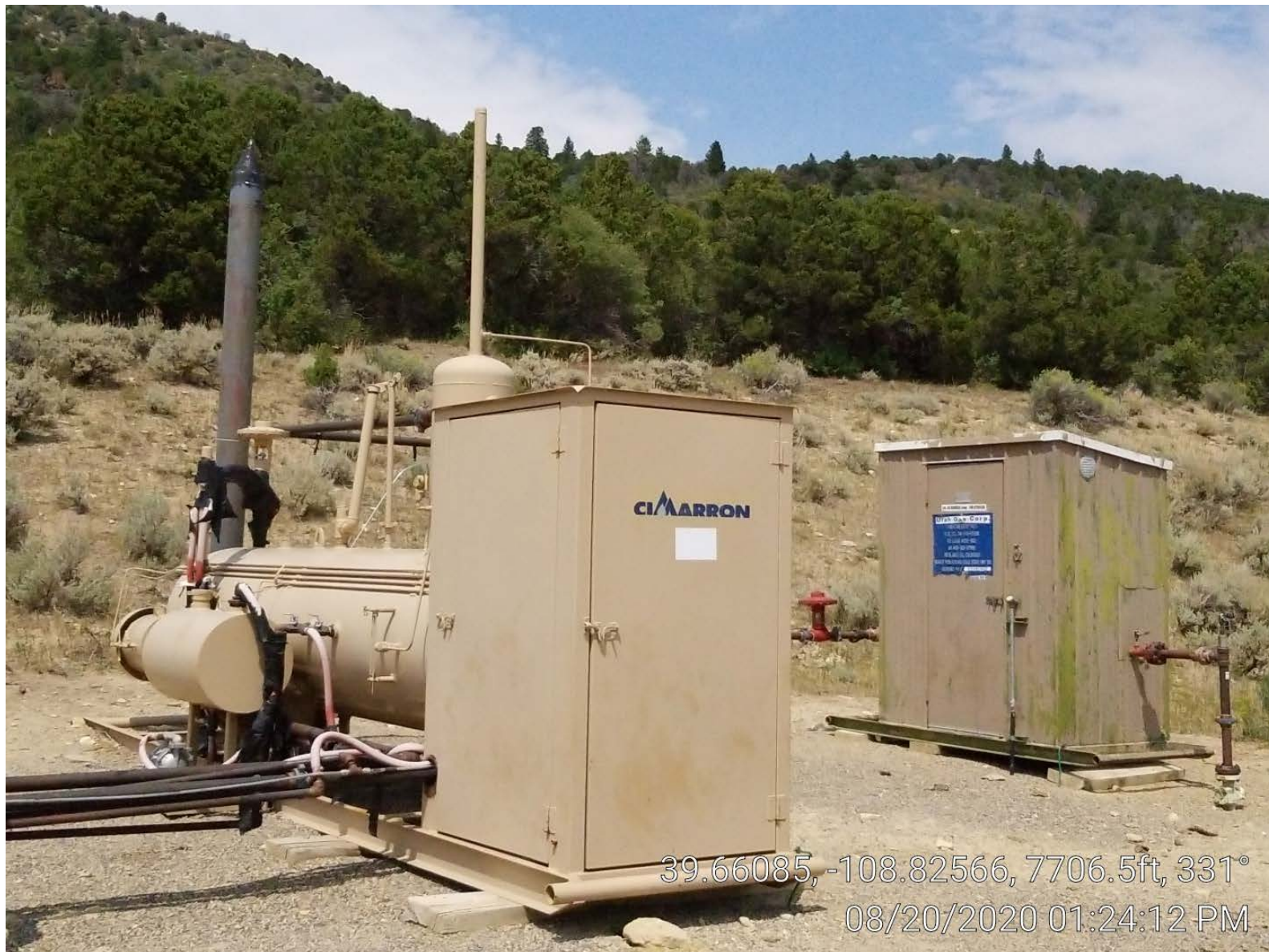
Photo 2. Separator & meter building.
