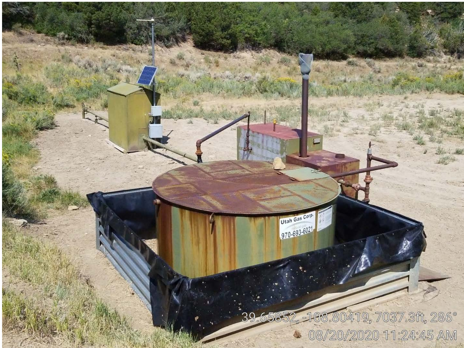
Photo 2. Tank, separator, meter building.
