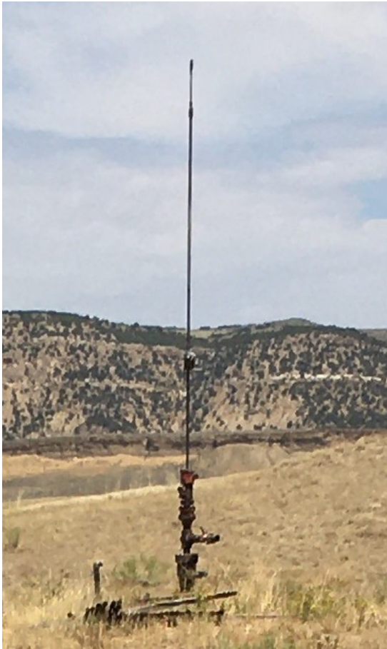
Wellhead with Polished rod installed in wellhead
