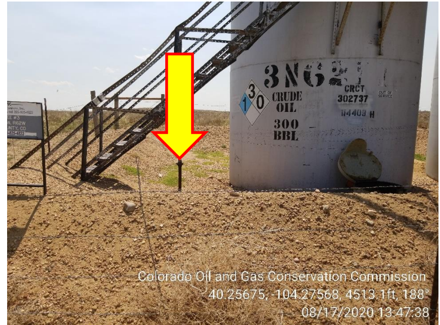
Photo – Unmarked Riser at Crude Oil Tanks
