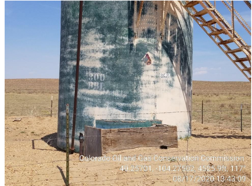
Photo 2 – Produced Water Tank – Content, Capacity and NFPA Labels have faded
