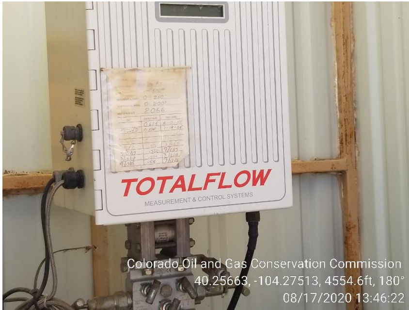
Photo 3 – Gas Meter appears not be updated on Calibration.
