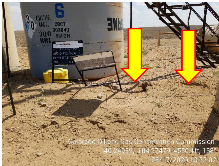
Photo 5 – Berms are inadequate
