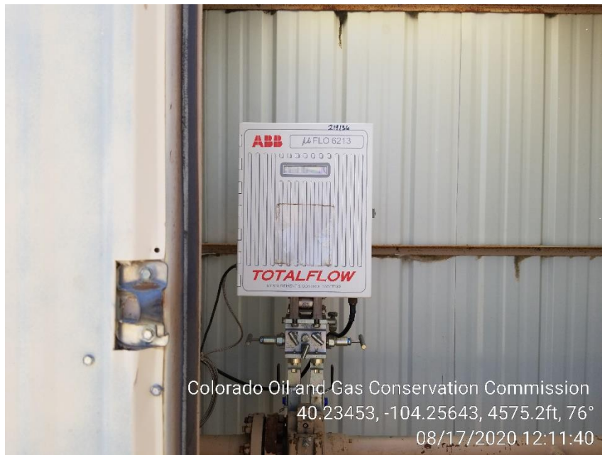
Photo 5 – Gas Meter, No Current Calibration card
