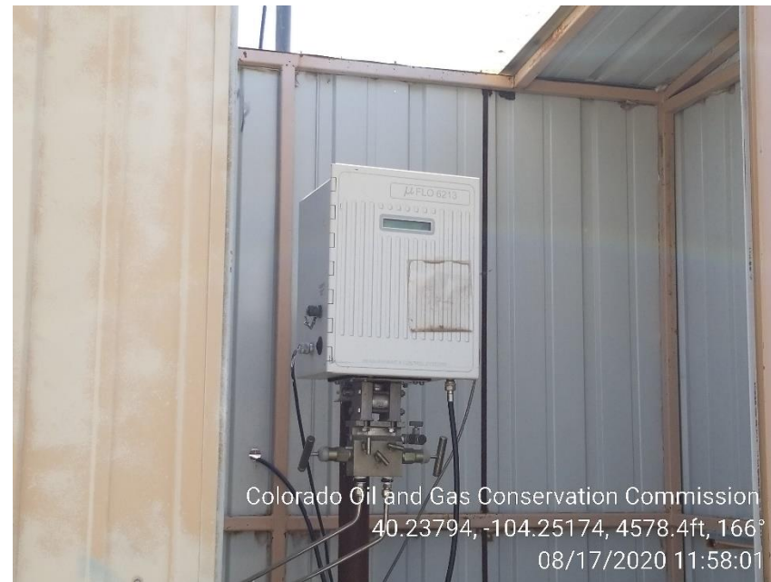
Photo 6 – Gas Meter, No Current Calibration card
