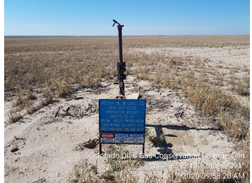
2. Pipeline riser still in place, (Tumbleweed Midstream)
