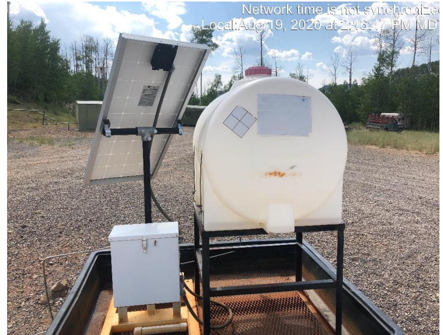
Photo #1759 Chemical tank not properly labeled.
