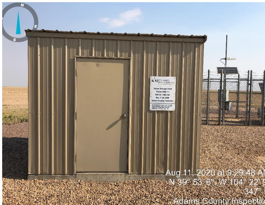
Photo #1 well house
