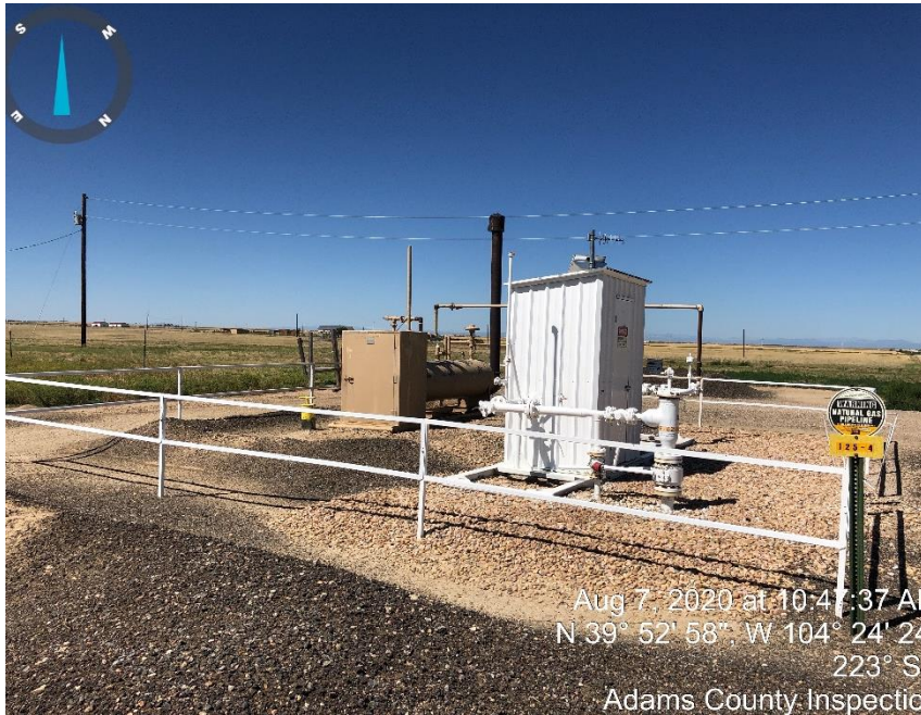
Photo #3 Meter & Separator.
