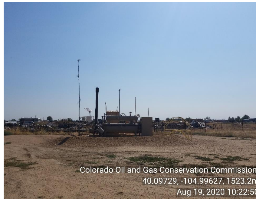
Photo 2 Meter house and separator
