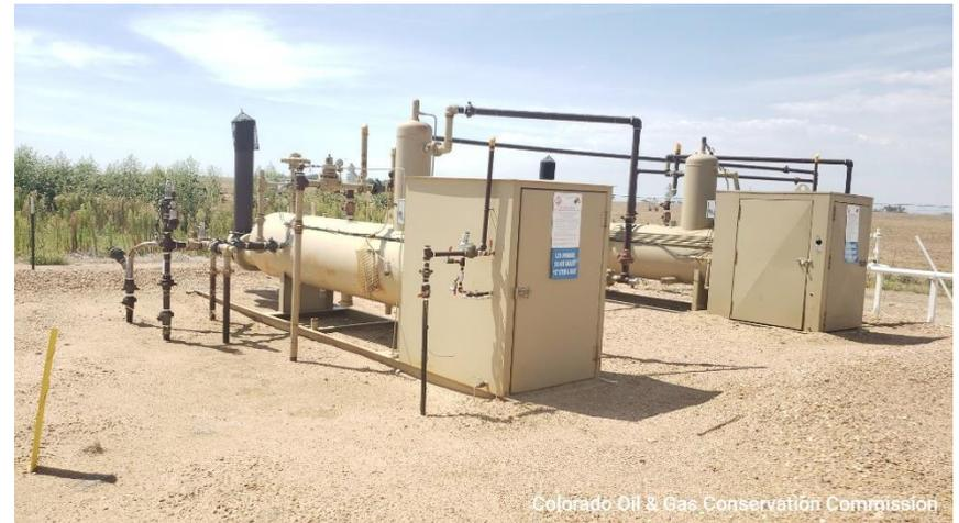
**Photo 6 Horizontal Heated Separators**
