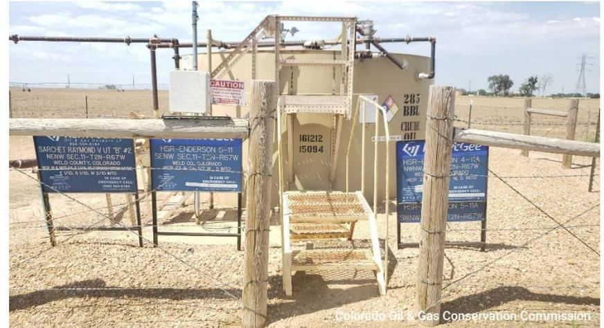
**Photo 7 Gas Meter Run, Door stuck closed on housing, Calibration is unknown at time of inspection.**
