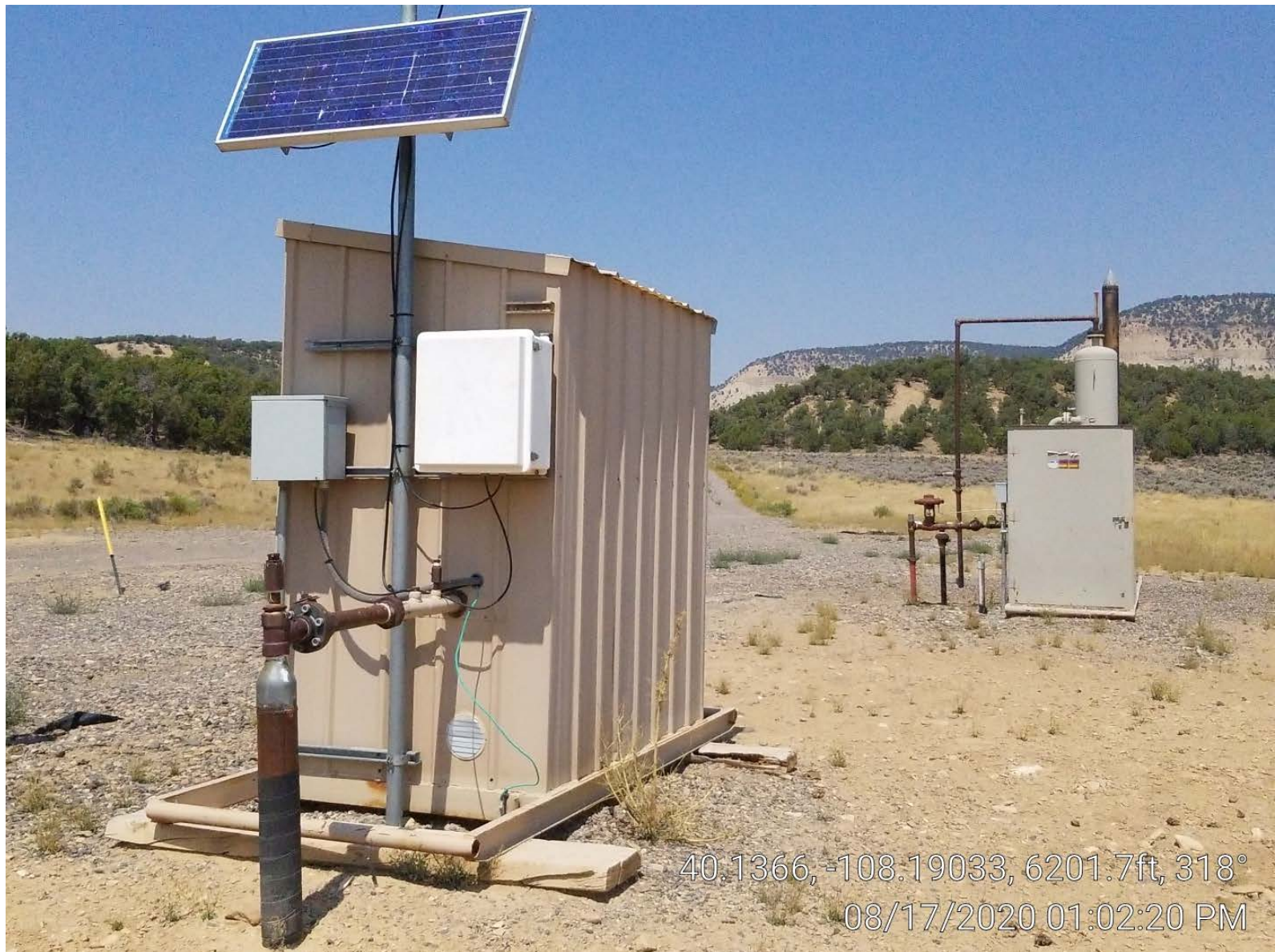
Photo 3. Meter building & separator.
