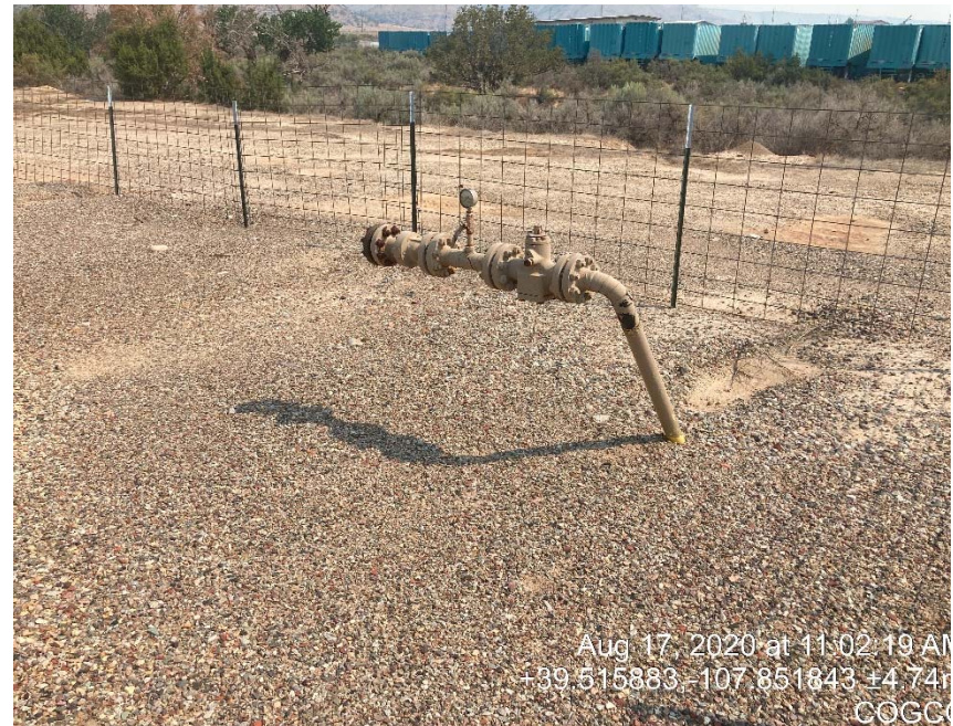
Unmarked flow line/ unused equipment
