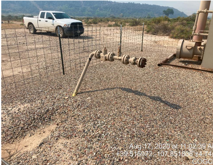
Unmarked flow line/ unused equipment
