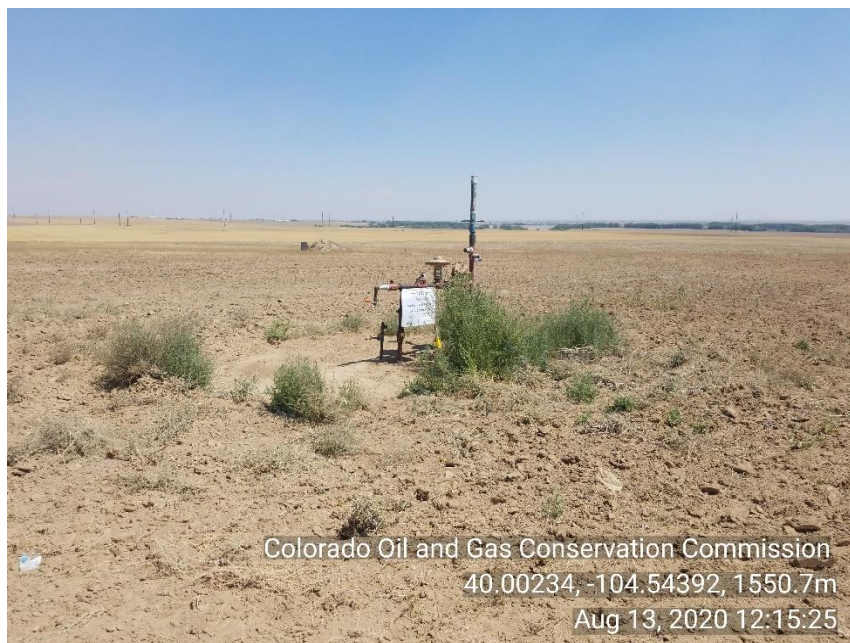
Photo 1 WH Flow line valves appear to be closed. Weeds around well head
