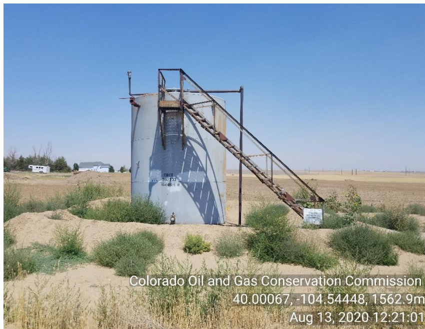
Photo 3 Crude oil tank. Weeds in and around containment. NFPA placards missing, no tank volume, Tank needs to be painted tank visible from county road.
