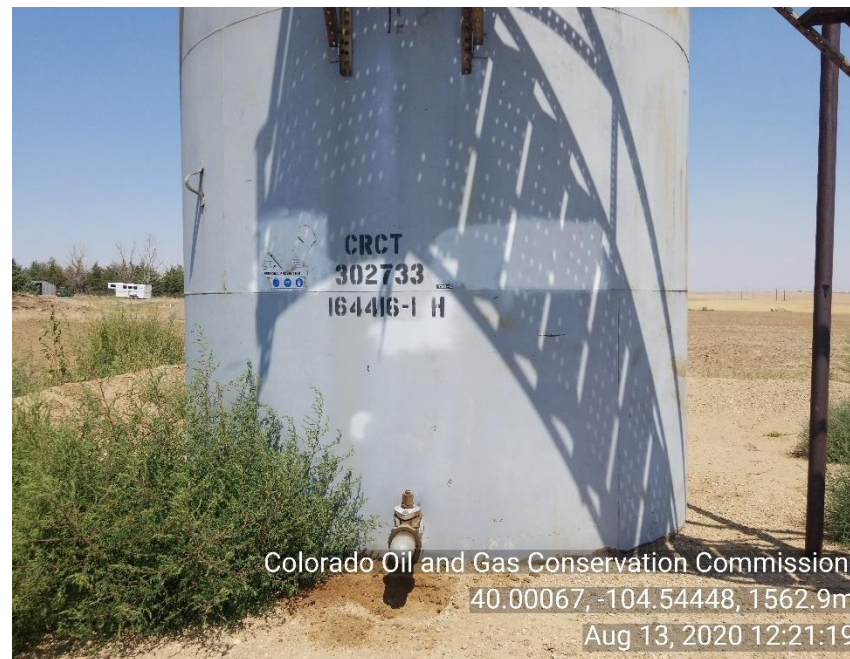
Photo 4 Stained soil under crude tank load out line. Mechanical issuer valve appears to be leaking. WEEDS
