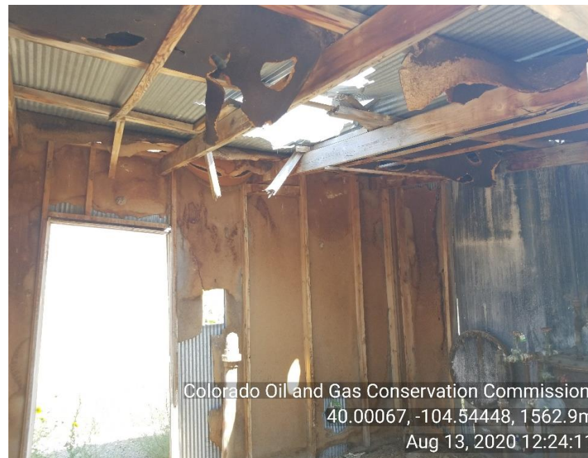
Photo 8 Vertical separator house in disrepair.
