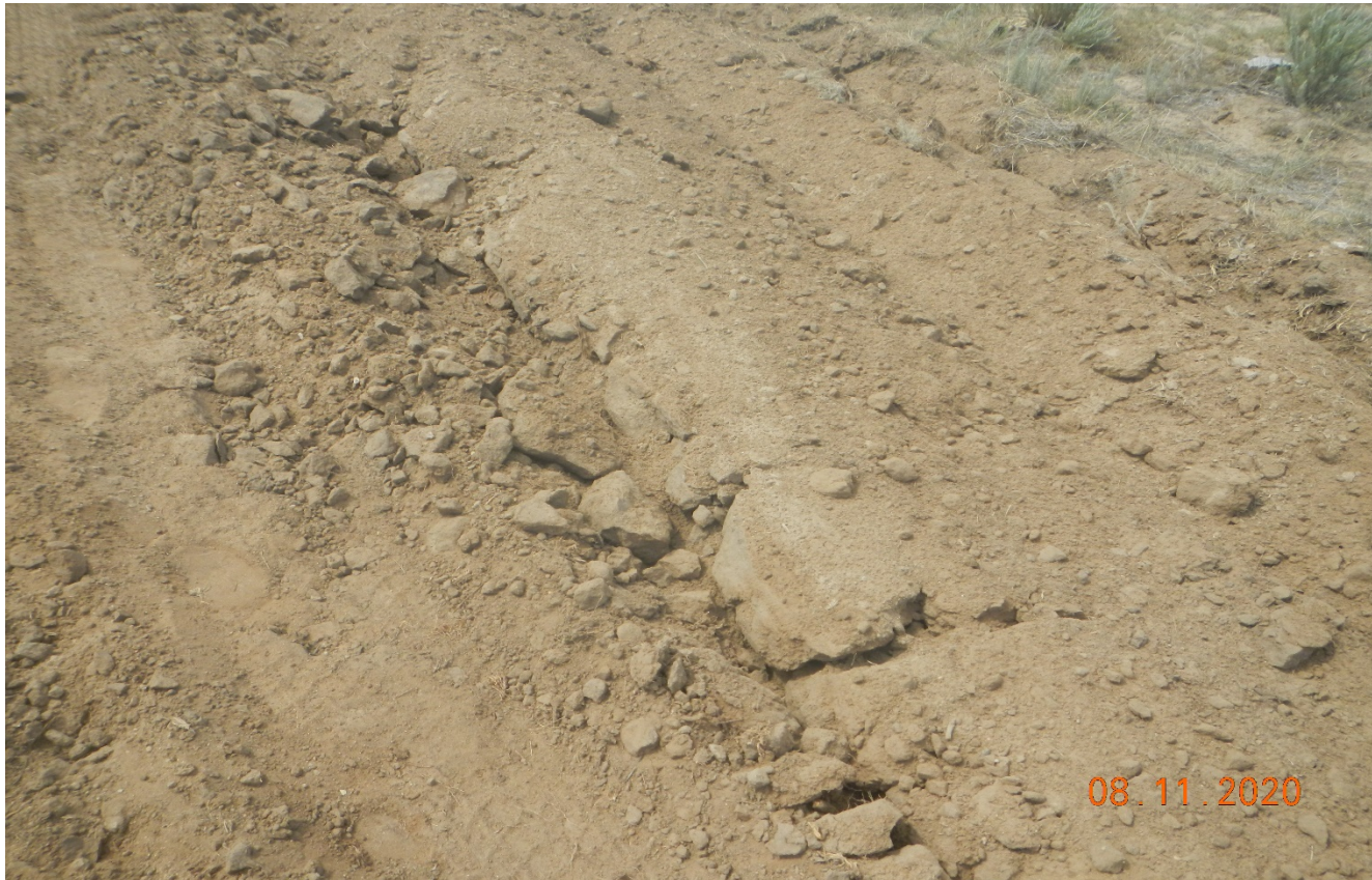
Photo 3. The soils were ripped but will need to be adequately tilled to establish a seed bed.
