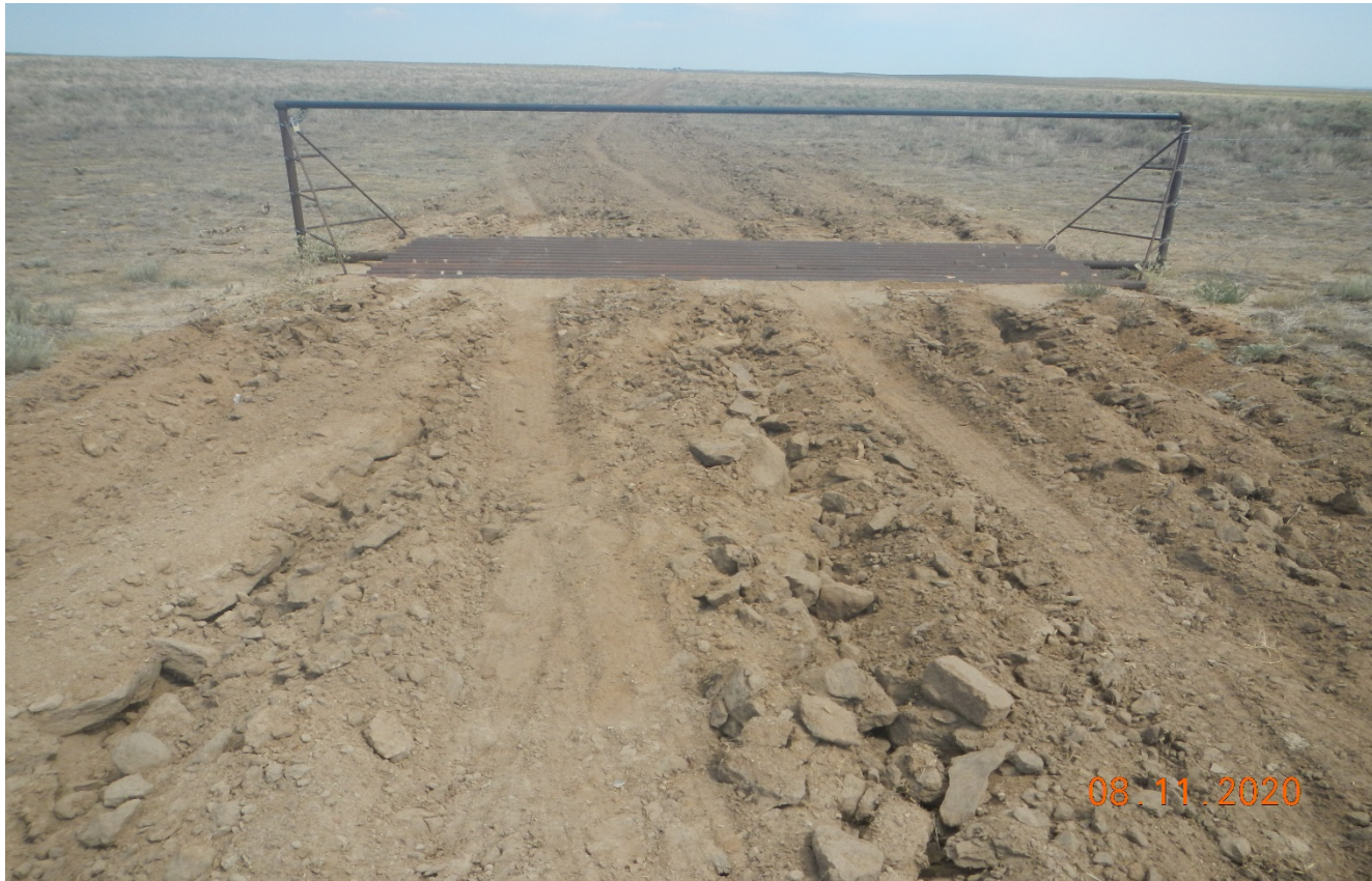
Photo 2. The soils were ripped along the access road. The cattle guard will need to be removed.
