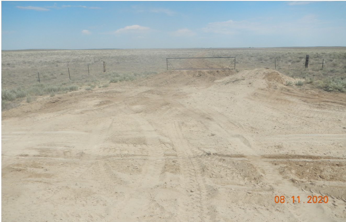
Photo 1. Facing north toward the beginning of the access road. The access from the county road has been regraded and soils decompacted.
