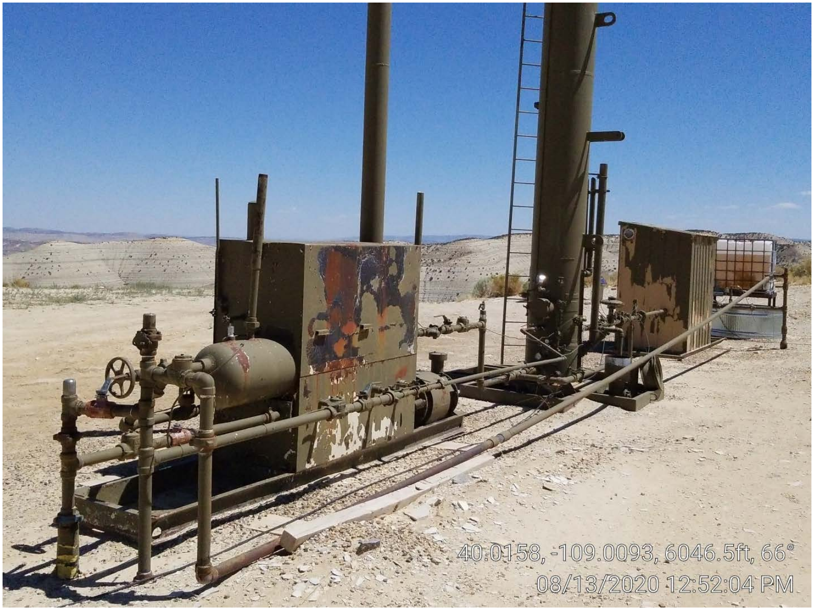
Photo 2. Separator & meter building.
