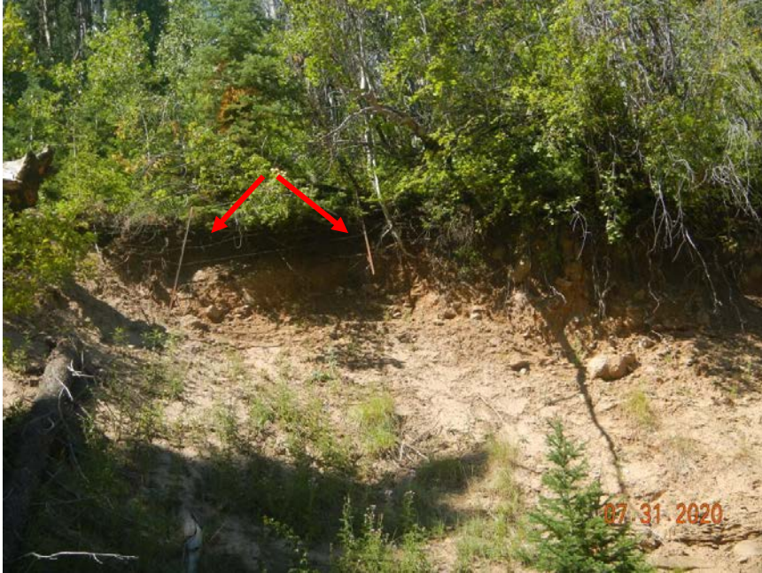
Photo#5: Erosion and undermining of root systems at top of Cut. Note undermined old fencing, indicated by arrows.
