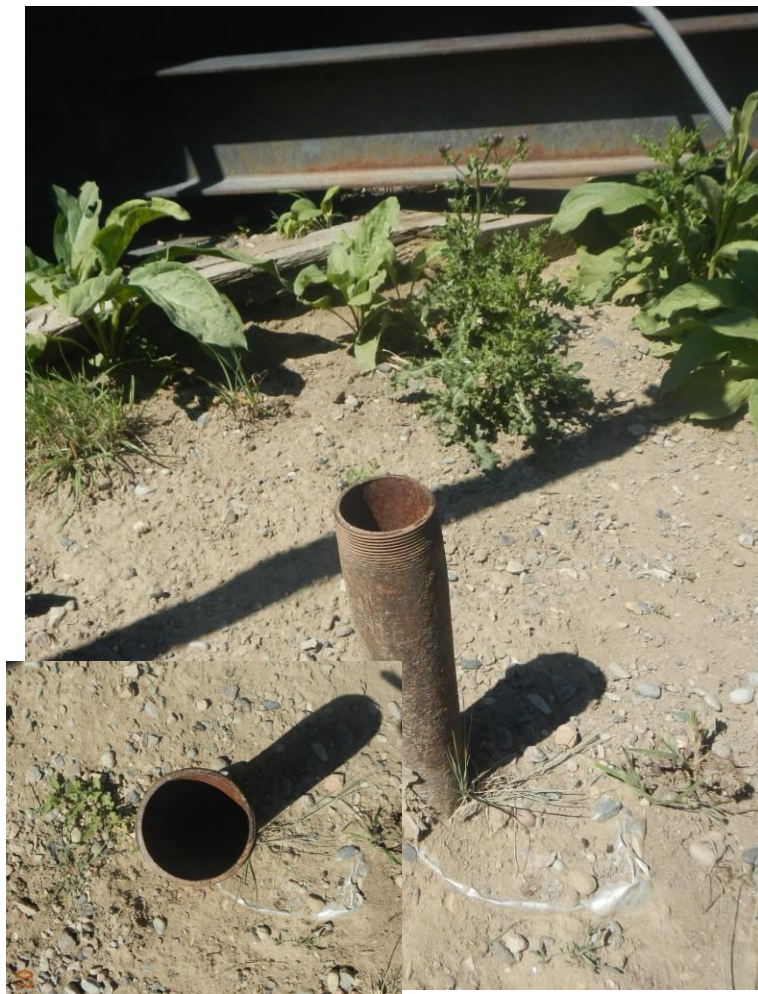
Photo#11: Open riser at front of Pump Jack.
