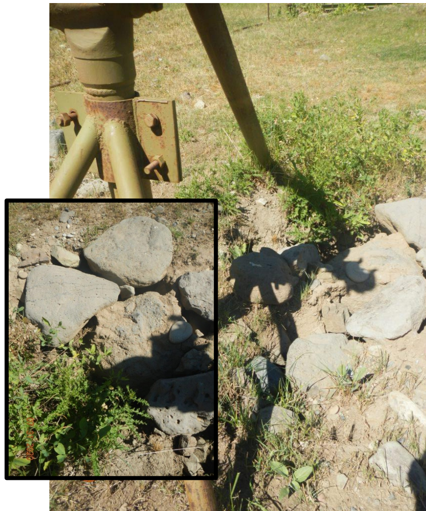
Photo#12: Subsidence/wormhole under rocked drain area.
