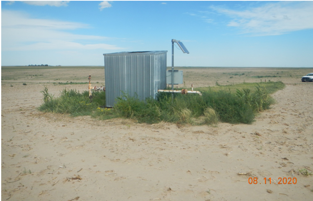
Photo 5. Facing northeast toward the meter shed. All equipment should have been removed within 3 months of plugging the well.
