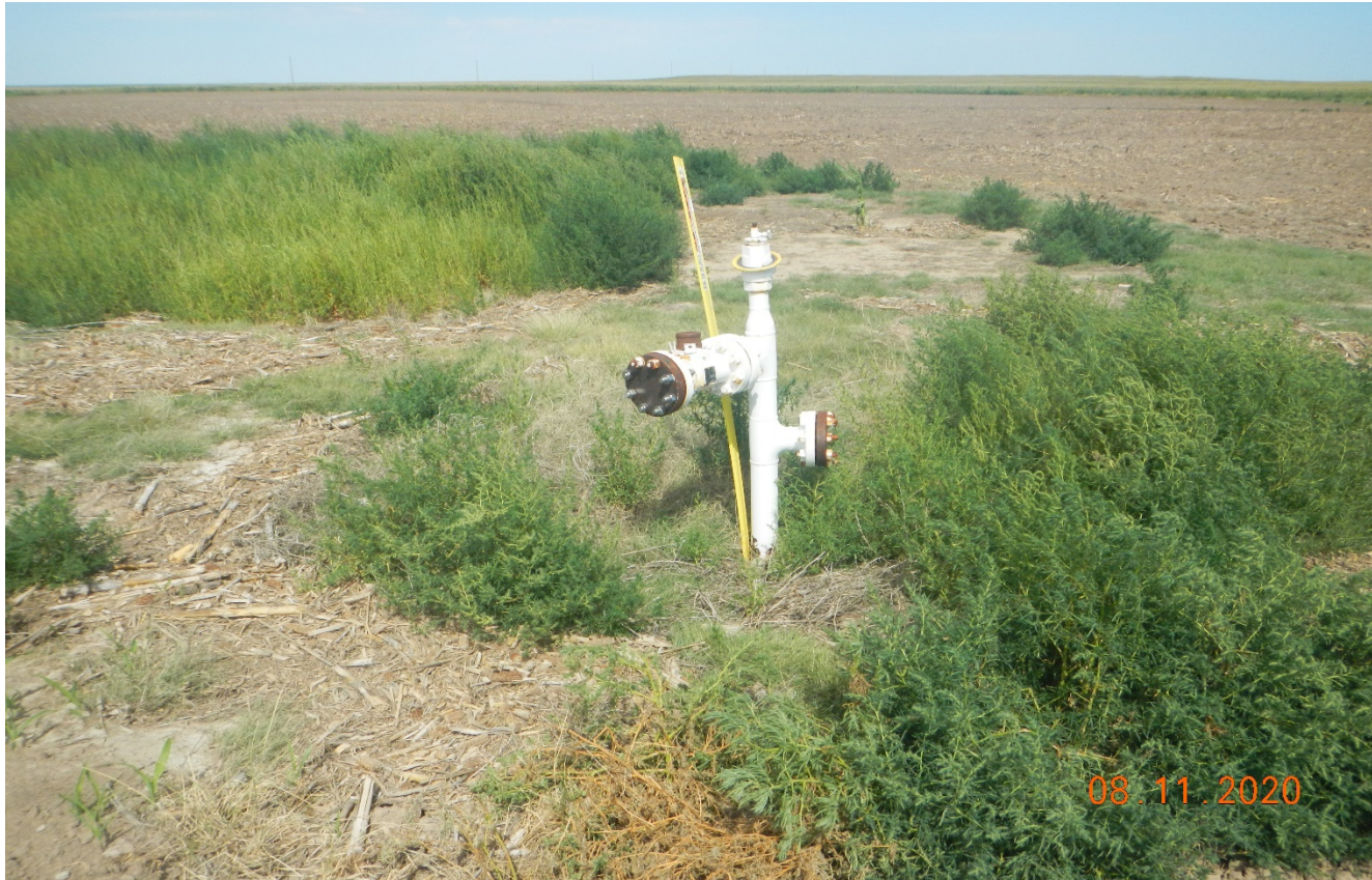
Photo 3. Pipe riser at the location has not been removed since previous inspection. Corrective action was not performed.
