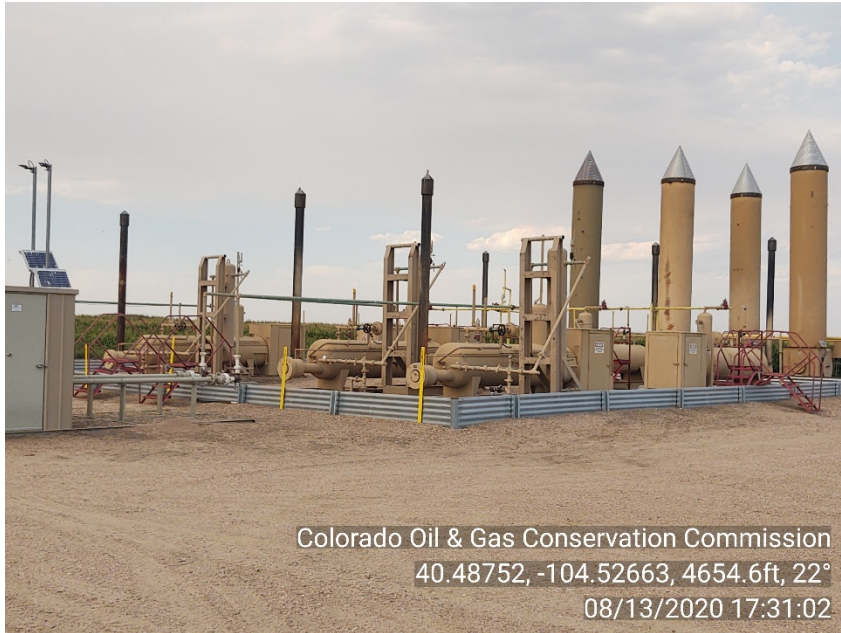
Photo #3 Rayglo A15-67-1HN, A15-68-1HN, Rayglo A14-67-1HN, A14-68-1HN Battery site: Separators Inactive | Shut-down
