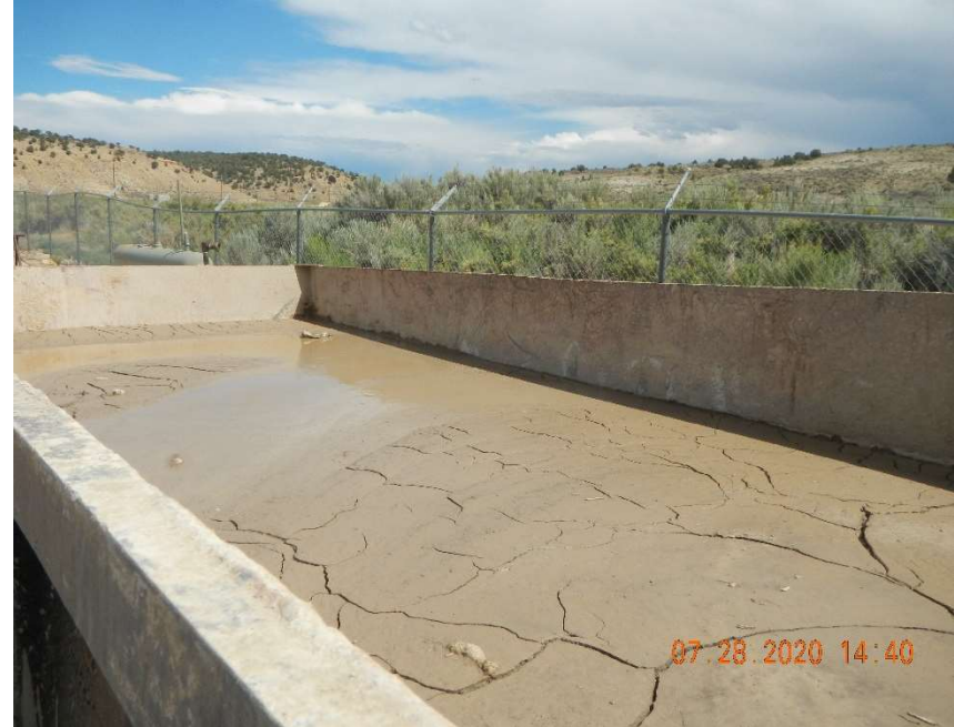
Stockpiled hydrovac material
