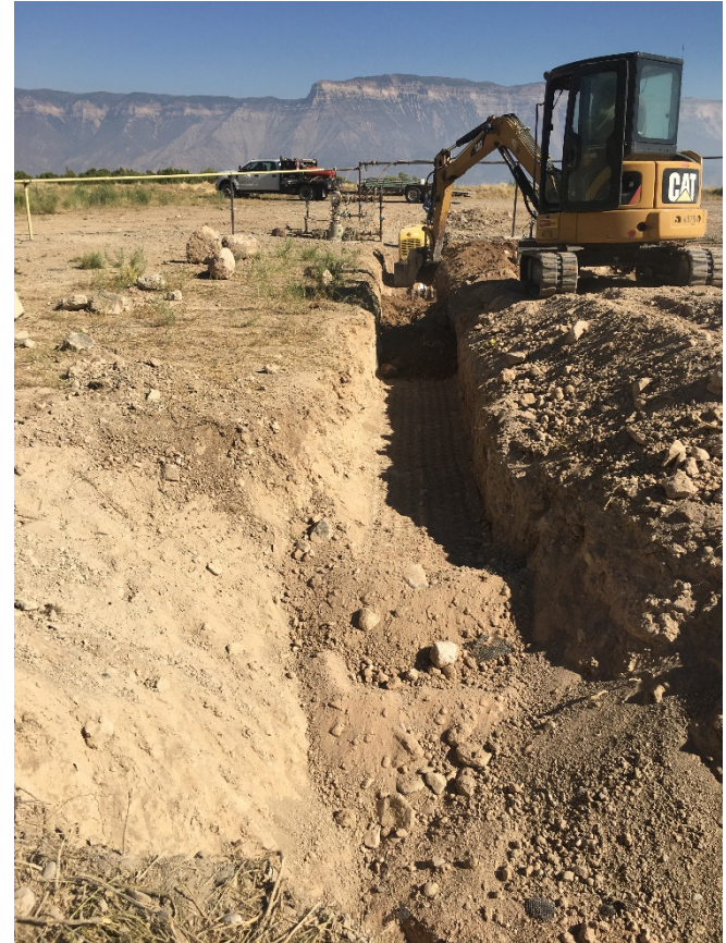
3" riser and flowline removed at wellhead and being compacted back fill
