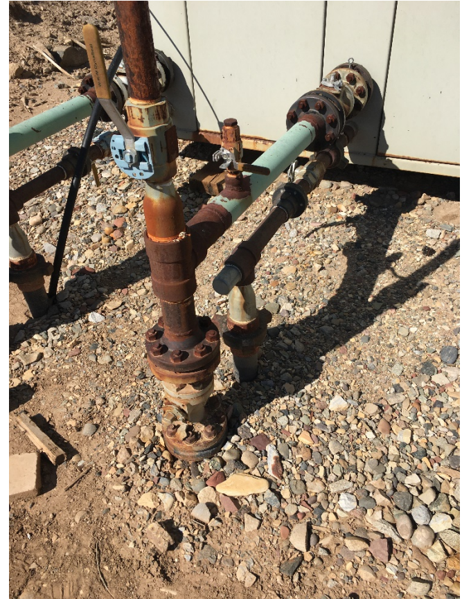
Two risers were left on the backside of separators; they are part of a active manifold system. Dump line and sales line
