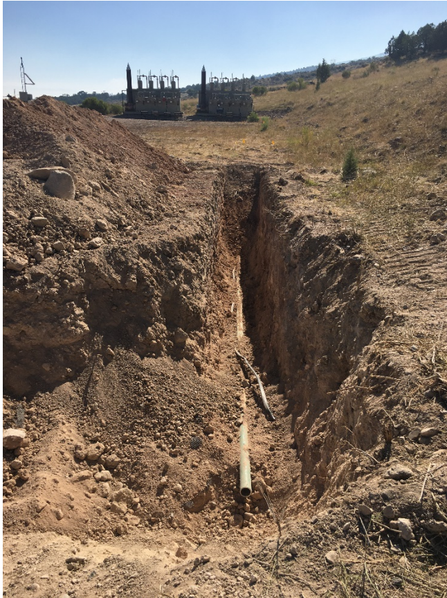
3" flowline from wellhead to separator in process of being removed
