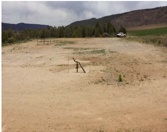
Date: 5/21/14 Picture: # 02 Description: Well Site after reclamation, looking south.
