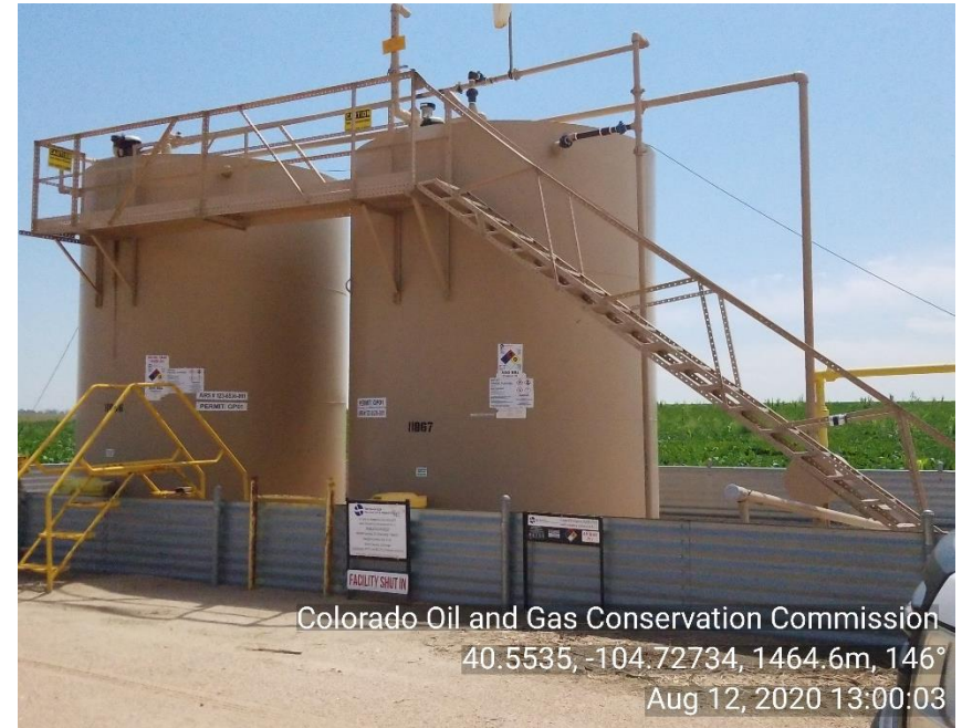
Photo 4: Tank Battery
