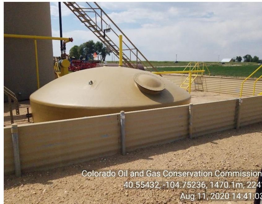
Photo 4: No labeling on tank
