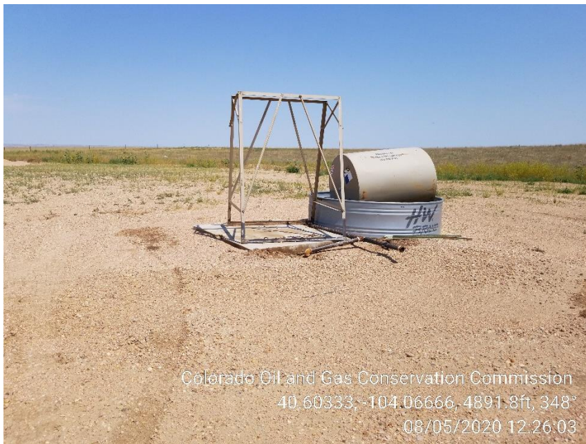
Photo 15 – Unused Chemical Tank and Containment, Stand
