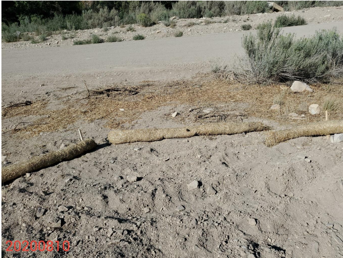
Photo 6: Continued from photo 5. Photo shows BMPs have not been installed in accordance with good engineering practices, and are not in proper functioning condition.
