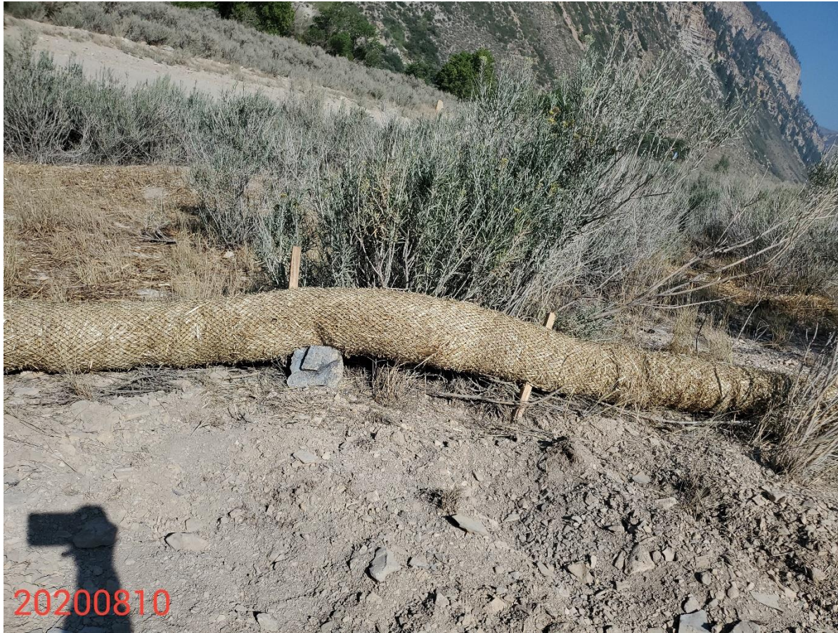
Photo 7: Continued from photo 5. Photo shows BMPs have not been installed in accordance with good engineering practices, and are not in proper functioning condition.
