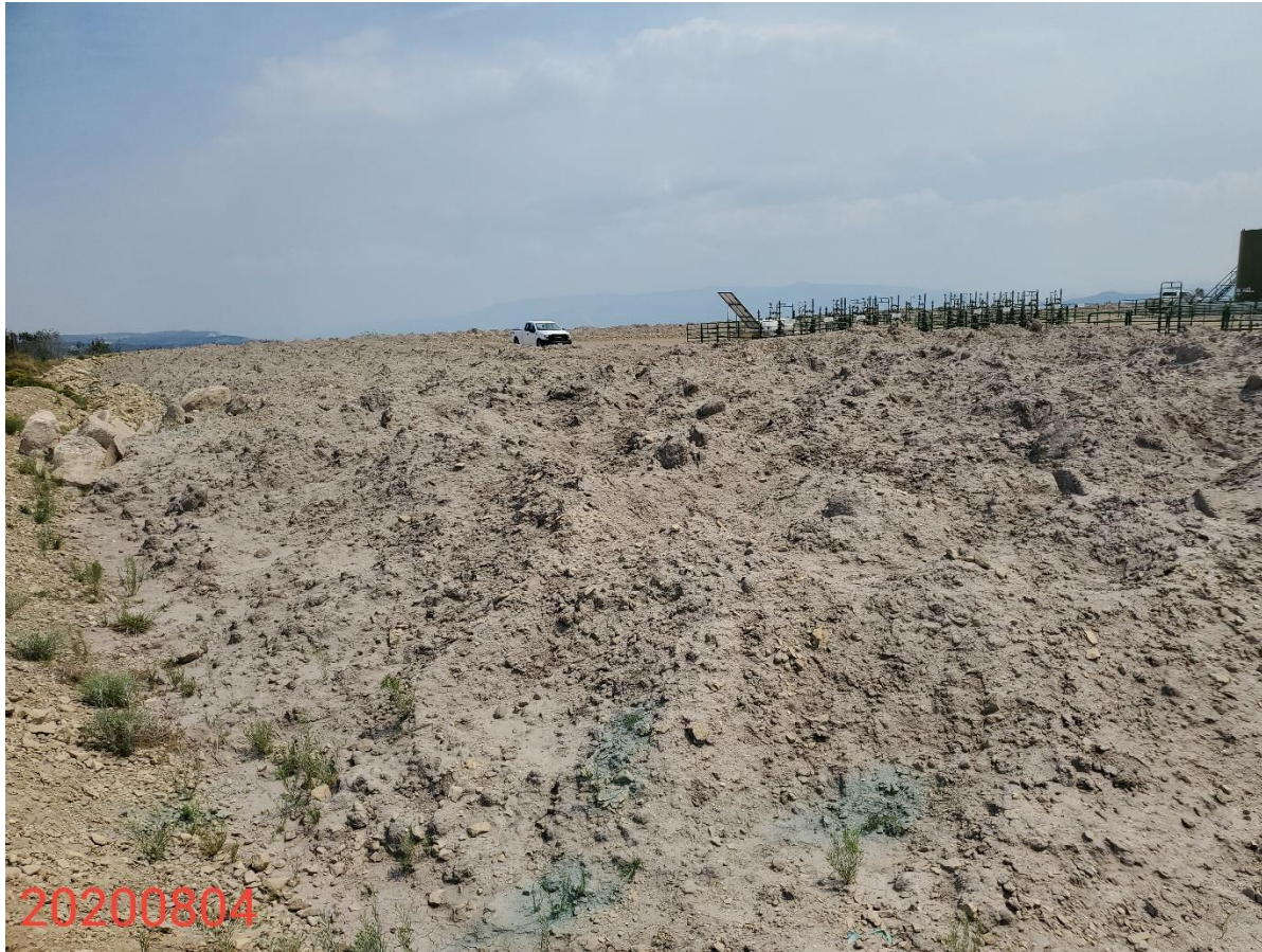
Photo 4: Photo taken from the northwest end of the Location, facing east. Photos 4-5 provide an overview of the Location from east to south. Photos also show drill cutting on the Location. Remediation project #11051 associated with cuttings management on the location was closed 10/2018; Interim reclamation of the Location has not been conducted.
