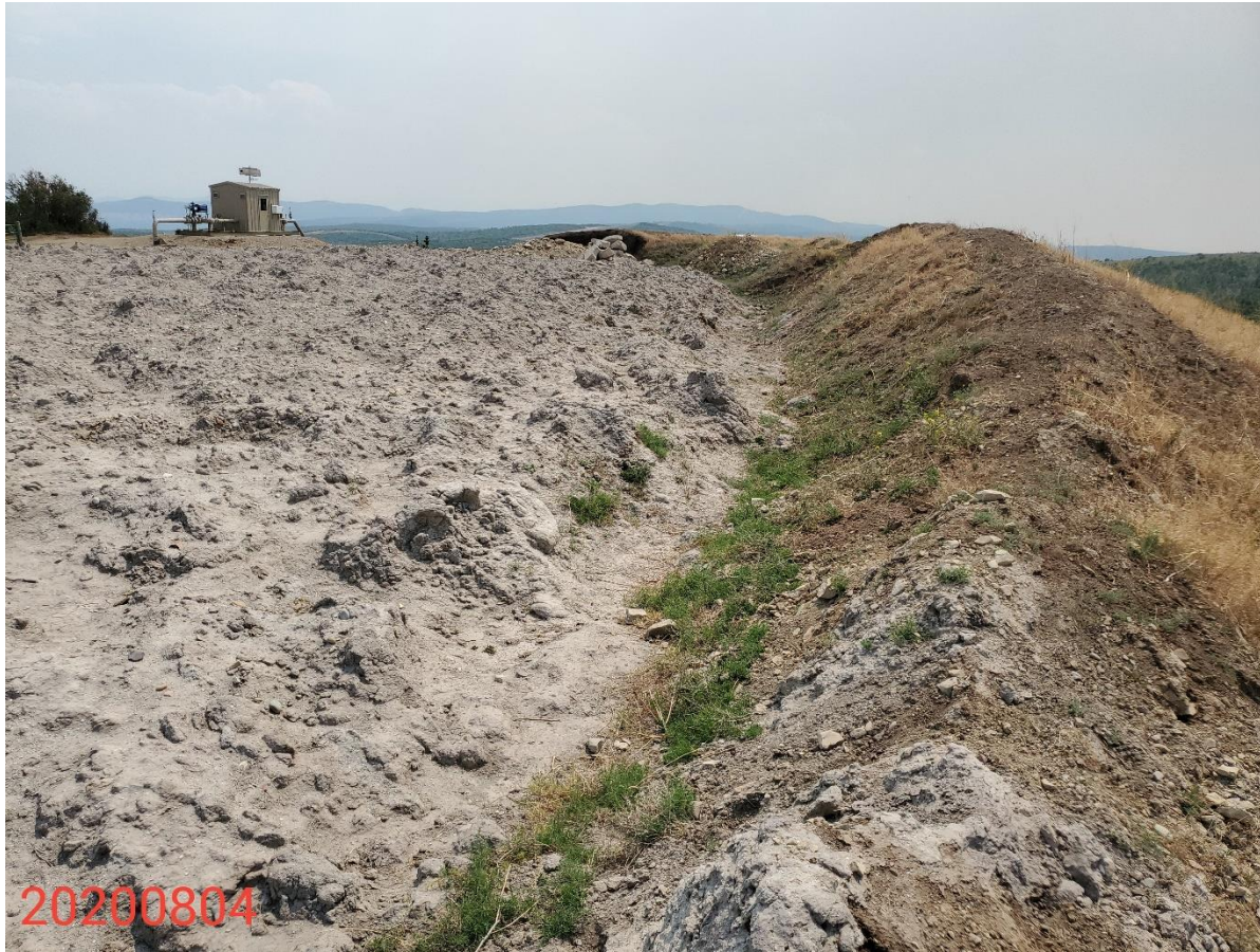
Photo 8: Photo taken from the west end of the Location, facing south. Photo shows topsoil stockpile and drill cuttings. There does not appear to be BMPs in place to segregate cuttings from the topsoil.
