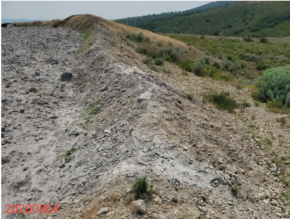
Photo 6: Photo taken from the west end of the Location, facing south. Photo shows areas where cuttings appear to have been pushed upon, and over the berm during management.
