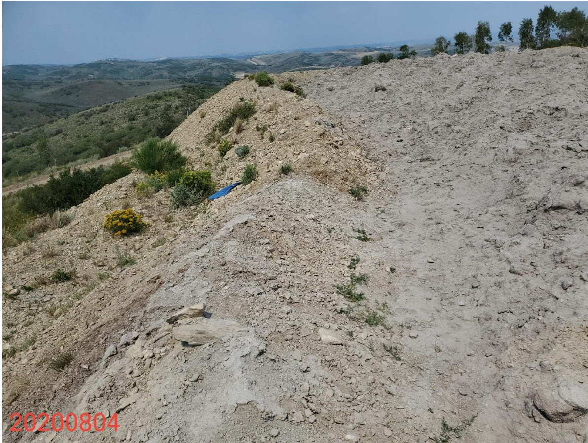
Photo 7: Photo taken from the west end of the Location, facing north. Photo shows areas where cuttings appear to have been pushed upon, and over the berm during management.
