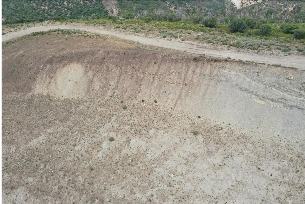
Photo 22: Aerial photo showing cut slopes on the north end of the Location, facing northwest. BMPs appear missing or insufficient to stabilize slopes. Interim areas have not been contoured/regraded and reclaimed to their original condition.
