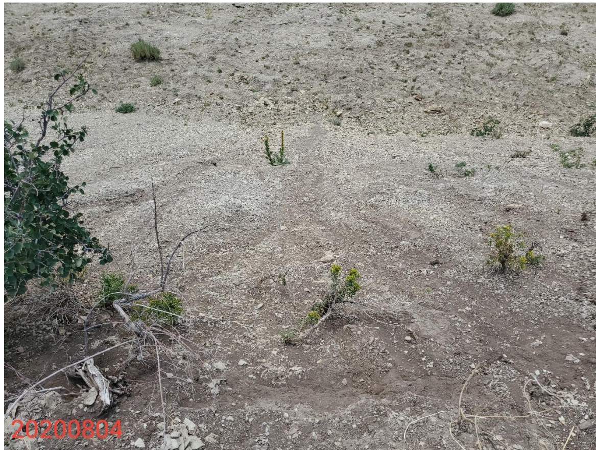
Photo 26: Photo taken from the cut slopes on the north end of the Location, facing south. BMPs appear missing or insufficient to stabilize slopes.
