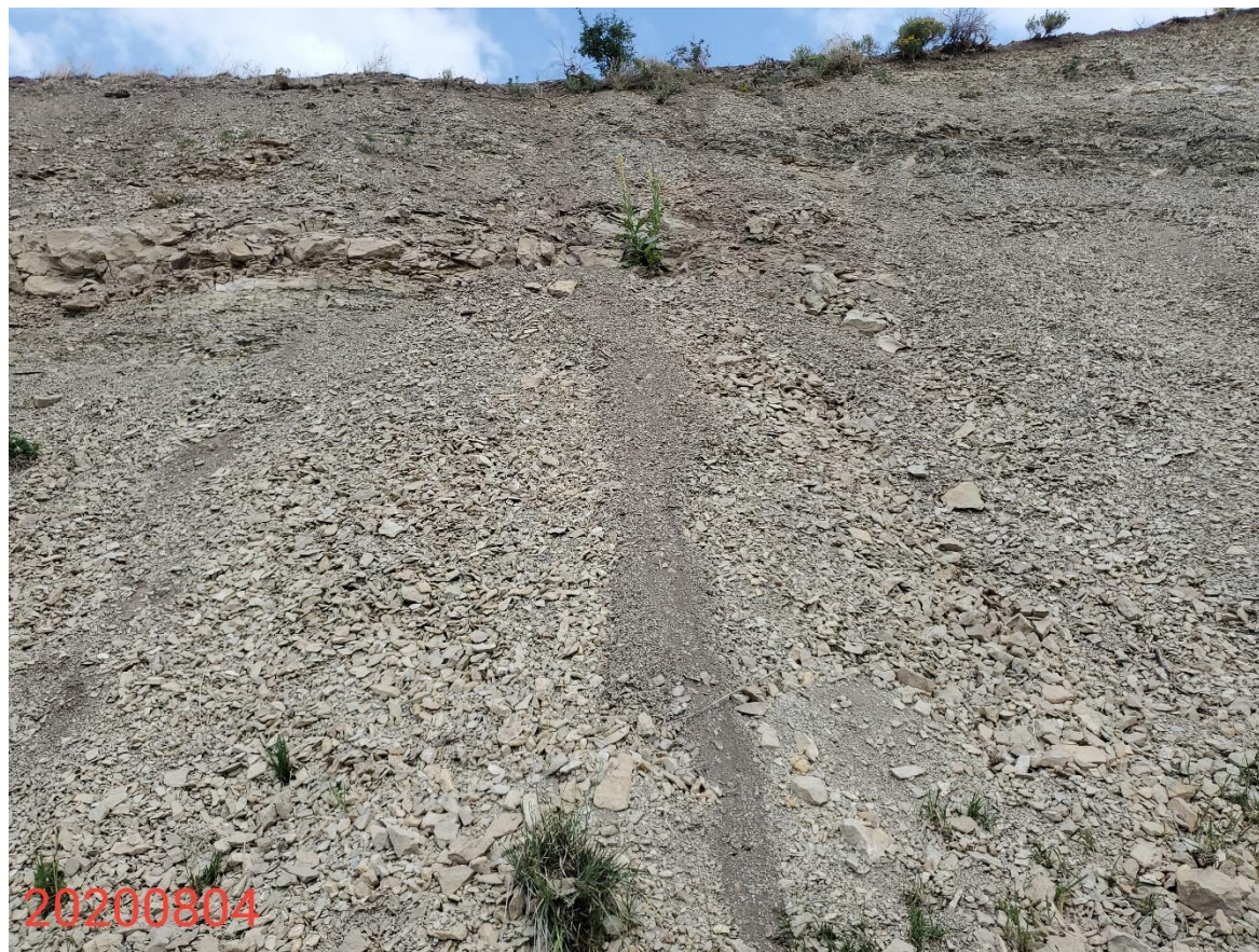
Photo 28: Photo taken from the northern interim areas, facing north. BMPs appear missing or insufficient to stabilize slopes.
