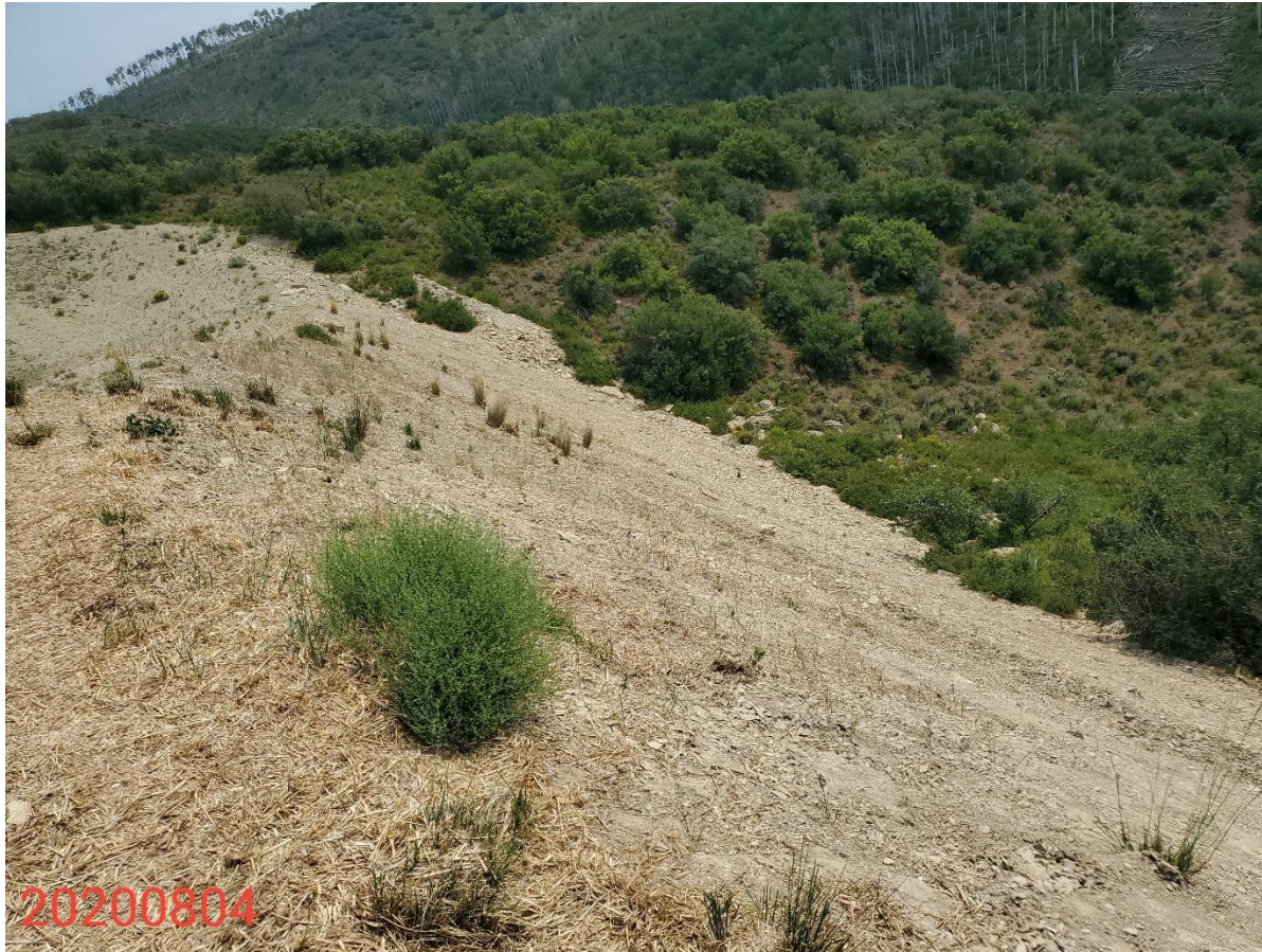
Photo 6: Photo taken from the southeast end of the Location, facing east. Photo shows areas of the Location, including fill slopes, that have not been recontoured/regraded or reclaimed to their original condition in accordance with 1003 rules. BMPs appear insufficient or missing to stabilize slopes and prevent sediment transport.
