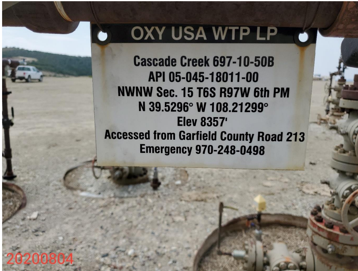
Photo 2: Continued from photo #1. Photo shows well with incorrect Operator information.
