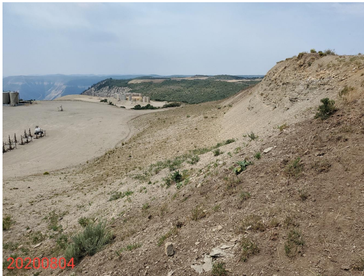
Photo 24: Photo taken from the northeast end of the Location, facing south. Photo shows cut slopes and interim areas. Interim areas have not been contoured/regraded and reclaimed to their original condition.
