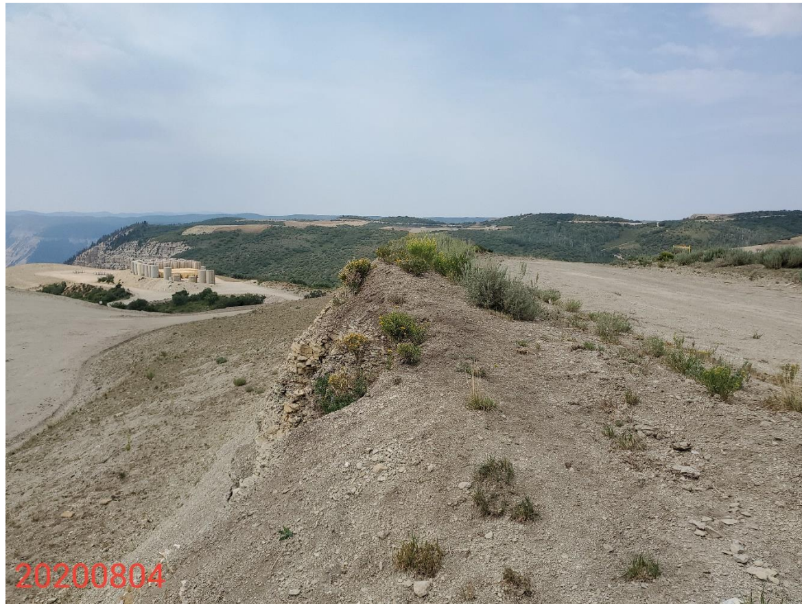
Photo 25: Photo taken from the northeast end of the Location, facing south. Photo shows cut slopes and interim areas. Interim areas do not appear to have been sufficiently recontoured/regraded and reclaimed to their original
