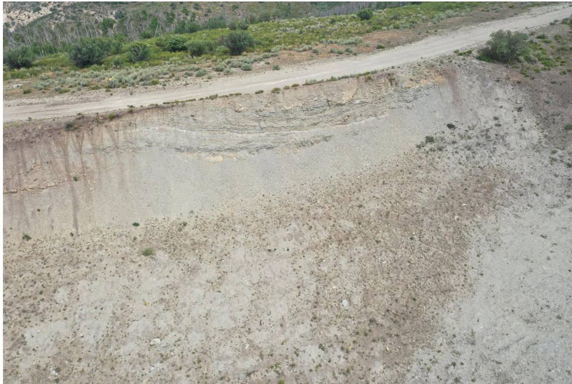
Photo 23: Aerial photo showing cut slopes on the north end of the Location, facing north. BMPs appear missing or insufficient to stabilize slopes. Interim areas have not been contoured/regraded and reclaimed to their original condition.
