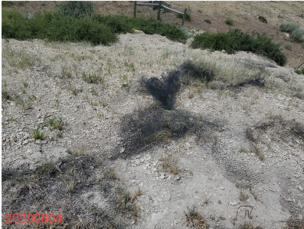
Photo 33: Photo of the slopes on the southwest end of the Location, facing south. Photo shows erosion net BMPs in disrepair.
