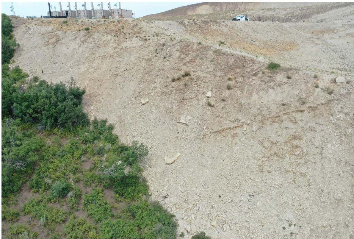
Photo 10: Photo taken from the south of the Location, facing northwest. Photo shows BMPs appear insufficient or missing to stabilize slopes and prevent sediment transport. Interim areas have not been contoured/regraded and reclaimed to their original condition.
