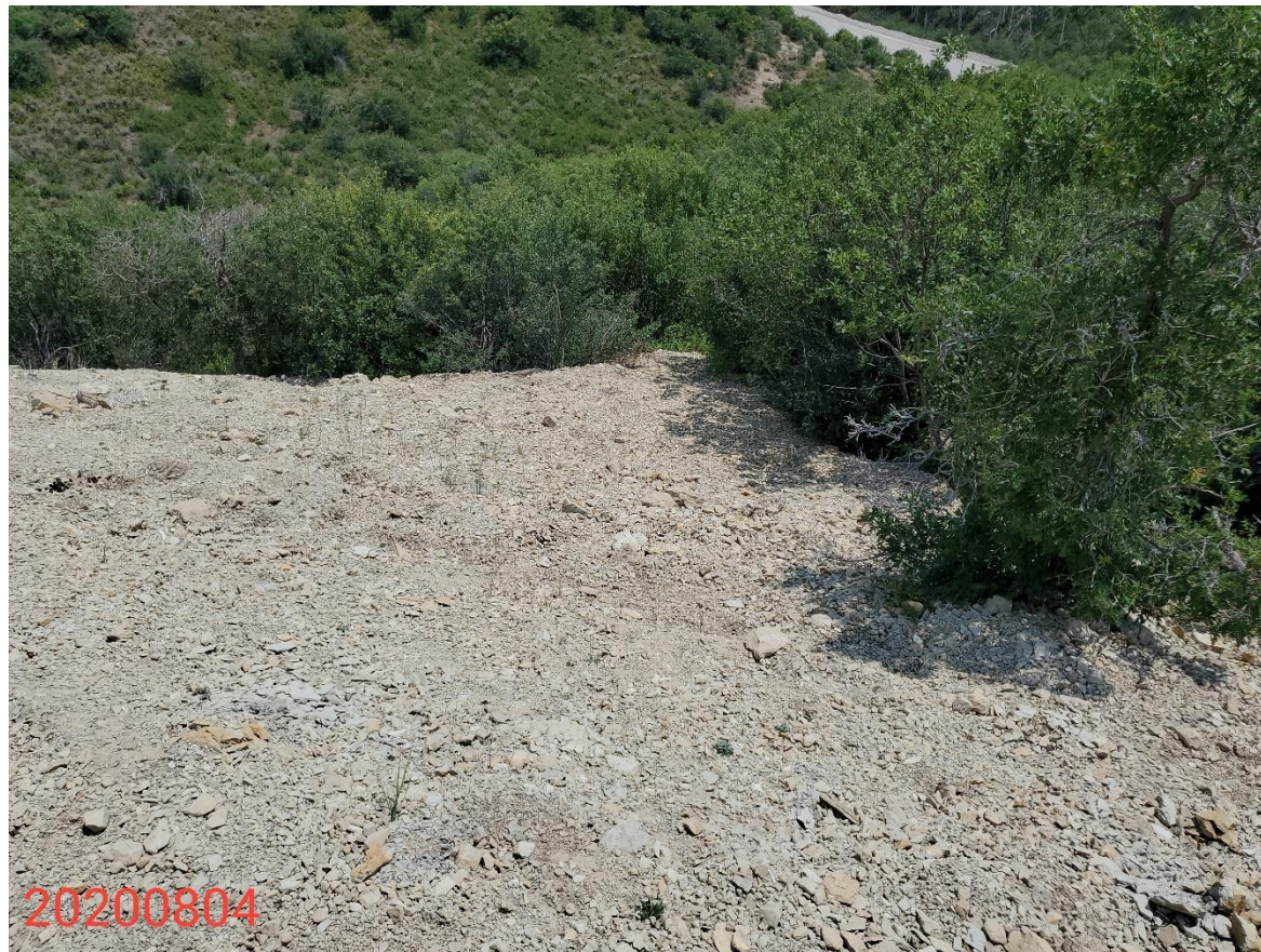
Photo 16: Photo taken from the eastern interim areas of the Location, facing east. Photo shows BMPs missing or insufficient to stabilize slopes and/or prevent sediment transport
