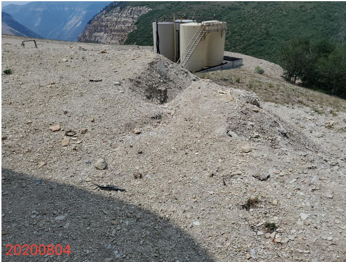
Photo 10: Photo taken from the southwestern end of the storage are of the location, facing southwest. Photo shows erosion degradation.
