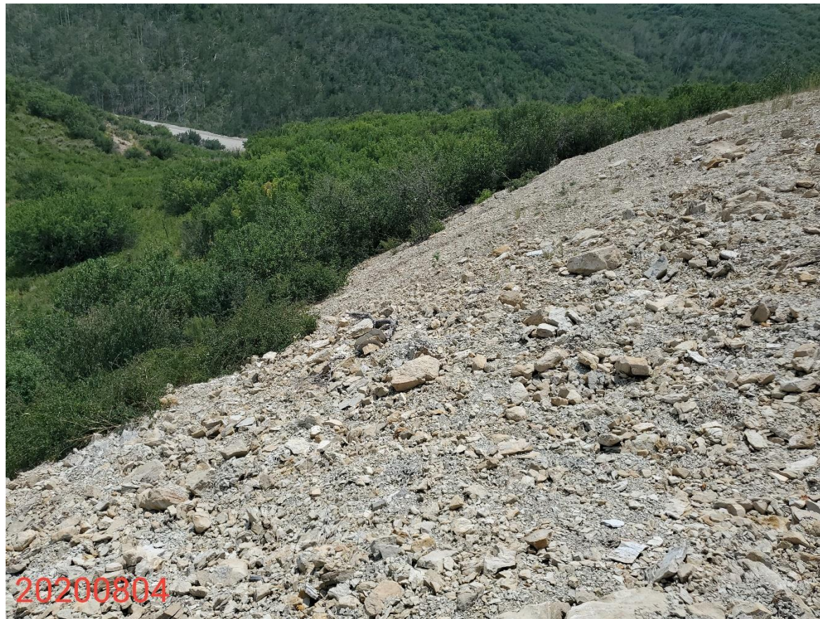
Photo 14: Photo taken from the eastern interim areas of the Location, facing southeast. Photo shows BMPs missing or insufficient to stabilize slopes and/or prevent sediment transport
