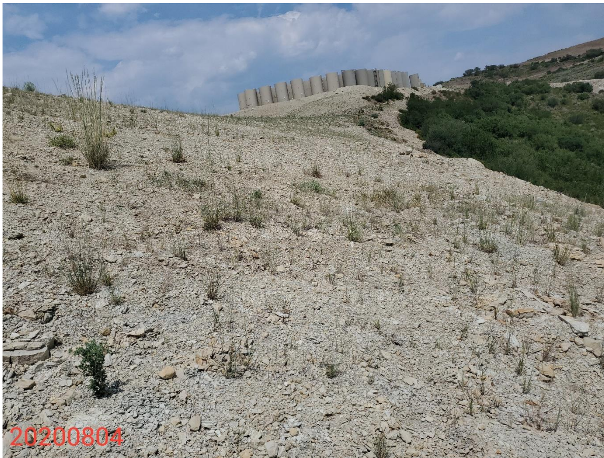
Photo 13: Photo taken from the eastern interim areas of the Location, facing north. Photo shows BMPs missing or insufficient to stabilize slopes and/or prevent sediment transport
