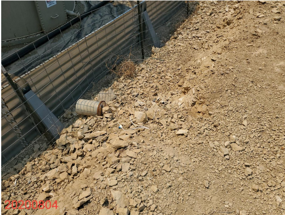
Photo 8: Photo taken from the northeast end of the tank battery. Photo shows what appears to be a part of a monitoring well; Well in disrepair. It is unclear if monitoring wells are needed for the Location and require maintenance to ensure proper functioning condition, or proper abandonment.
