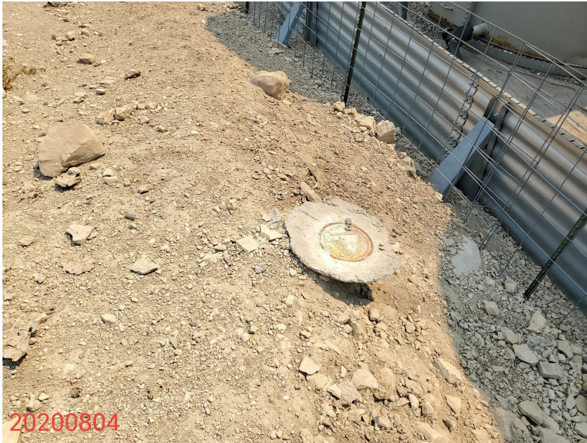
Photo 10: Photo taken from the northeast end of the tank battery. Photo shows second observed monitoring well. It is unclear if monitoring wells are needed for the Location and require maintenance to ensure proper functioning condition, or proper abandonment.
