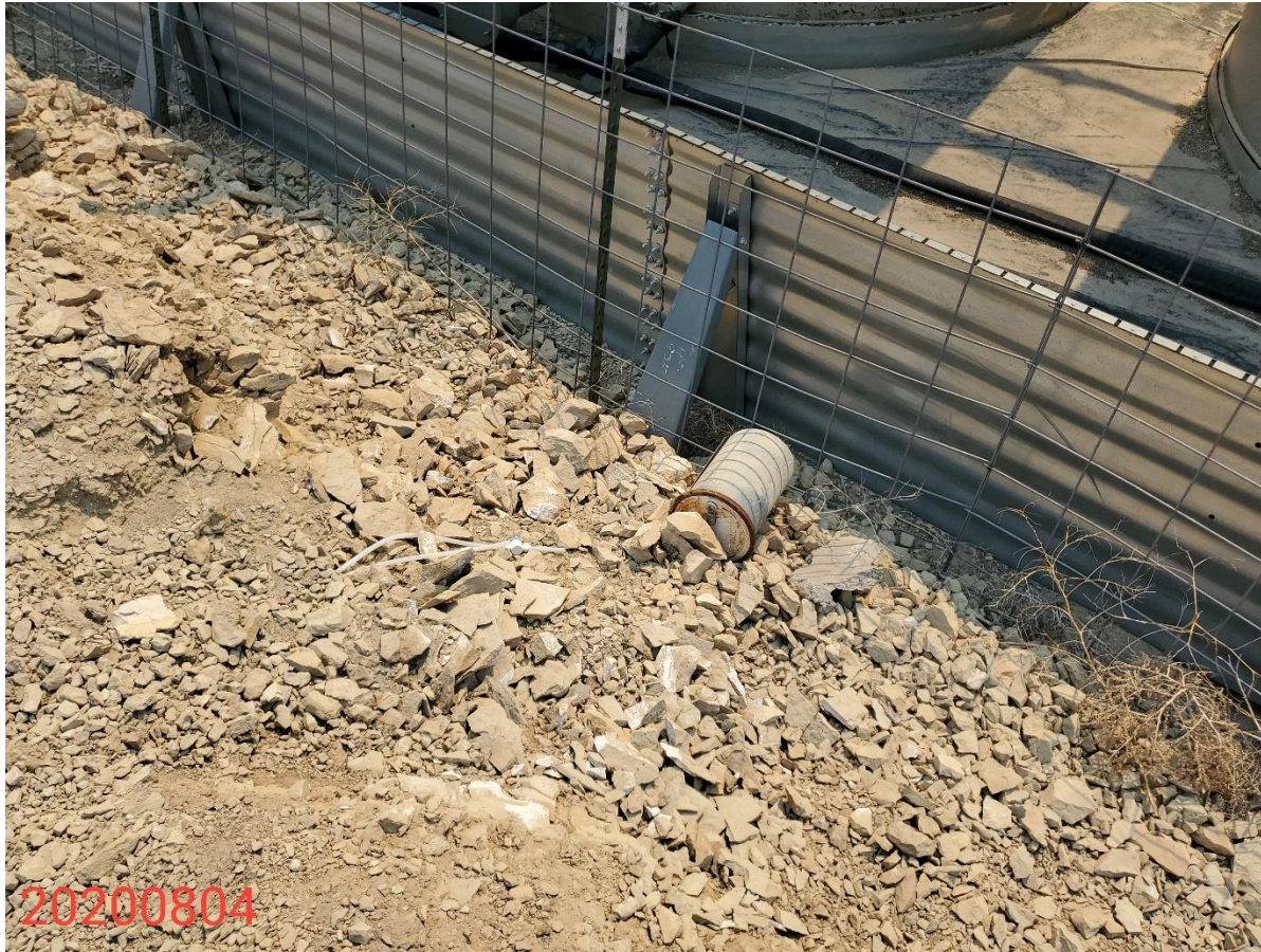
Photo 9: Continued from photo 8. Photo shows topsoil stockpile and drill cuttings. There does not appear to be BMPs in place to segregate cuttings from the topsoil.
