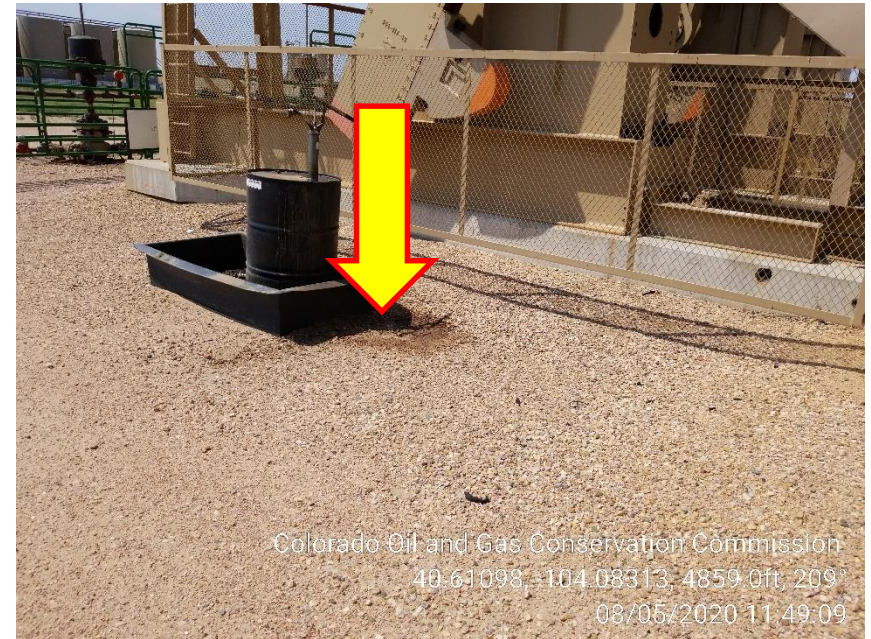
Photo 6 – Stained Soil at Chemical Tank
