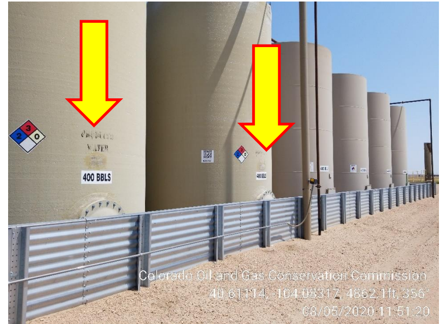
Photo 8 – South Tanks – Content and Capacity have faded no longer visible.
