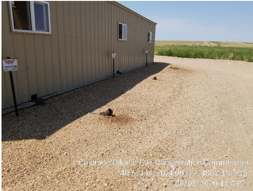
Photo 7 – Stained Soil at Exhaust
