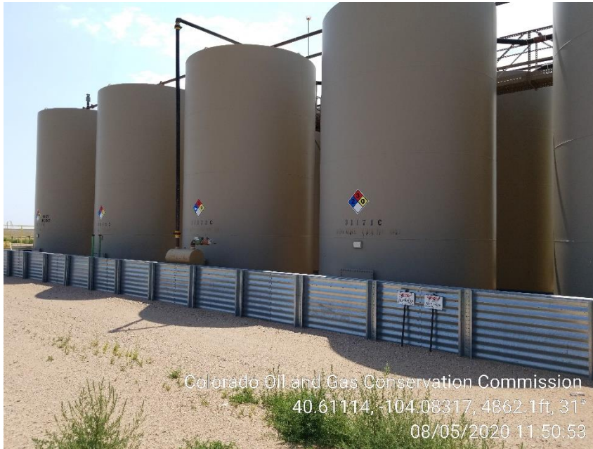
Photo 3 – North Tanks – Content and Capacity have faded no longer visible.
