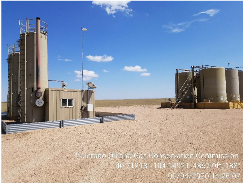
Photo 3 – Heater Treaters/Tank Battery
