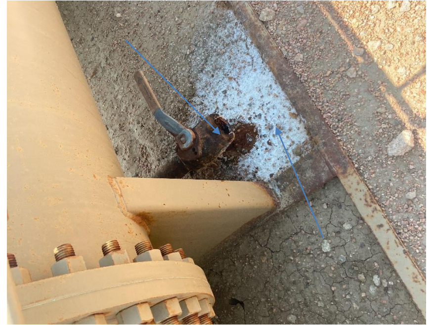
Pic 6 stained soil / mechanical issue
