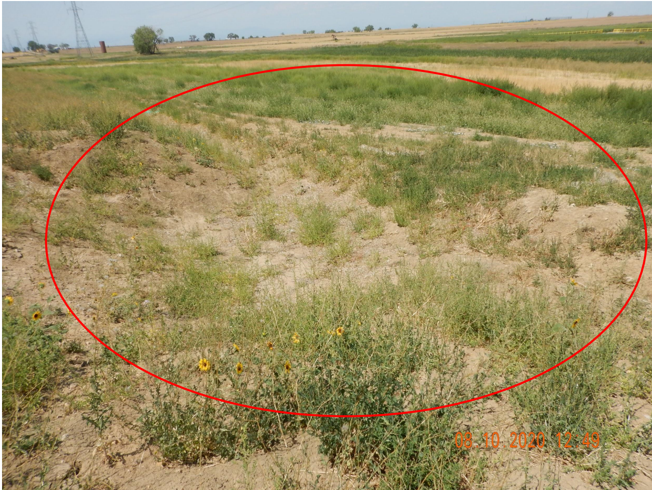
Photo 1. Photo taken from the northern location, facing Northwest. Photo illustrates a sediment trap stormwater BMP with a temporarily stabilized outlet. At the time of this inspection, BMPs appear to be in proper functioning condition. However, undesirable and noxious weed management is required. Refer to Photos 2-7 which also document weed management compliance issues.
