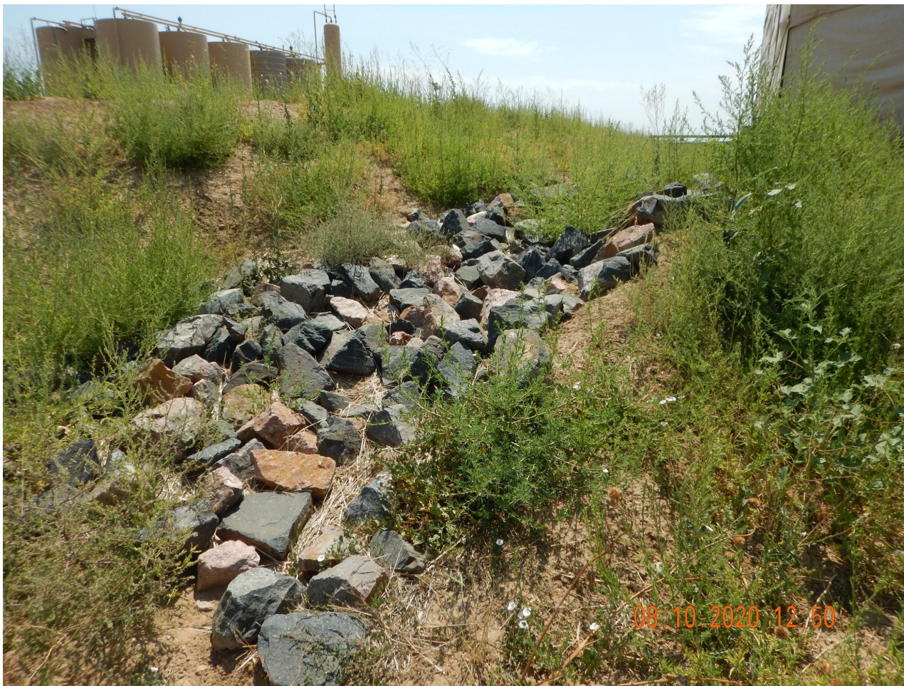
Photo 3. Photo taken from the northeastern location, facing South. Photo illustrates a stabilized diversion ditch which is directed to a temporarily stabilized outlet.
