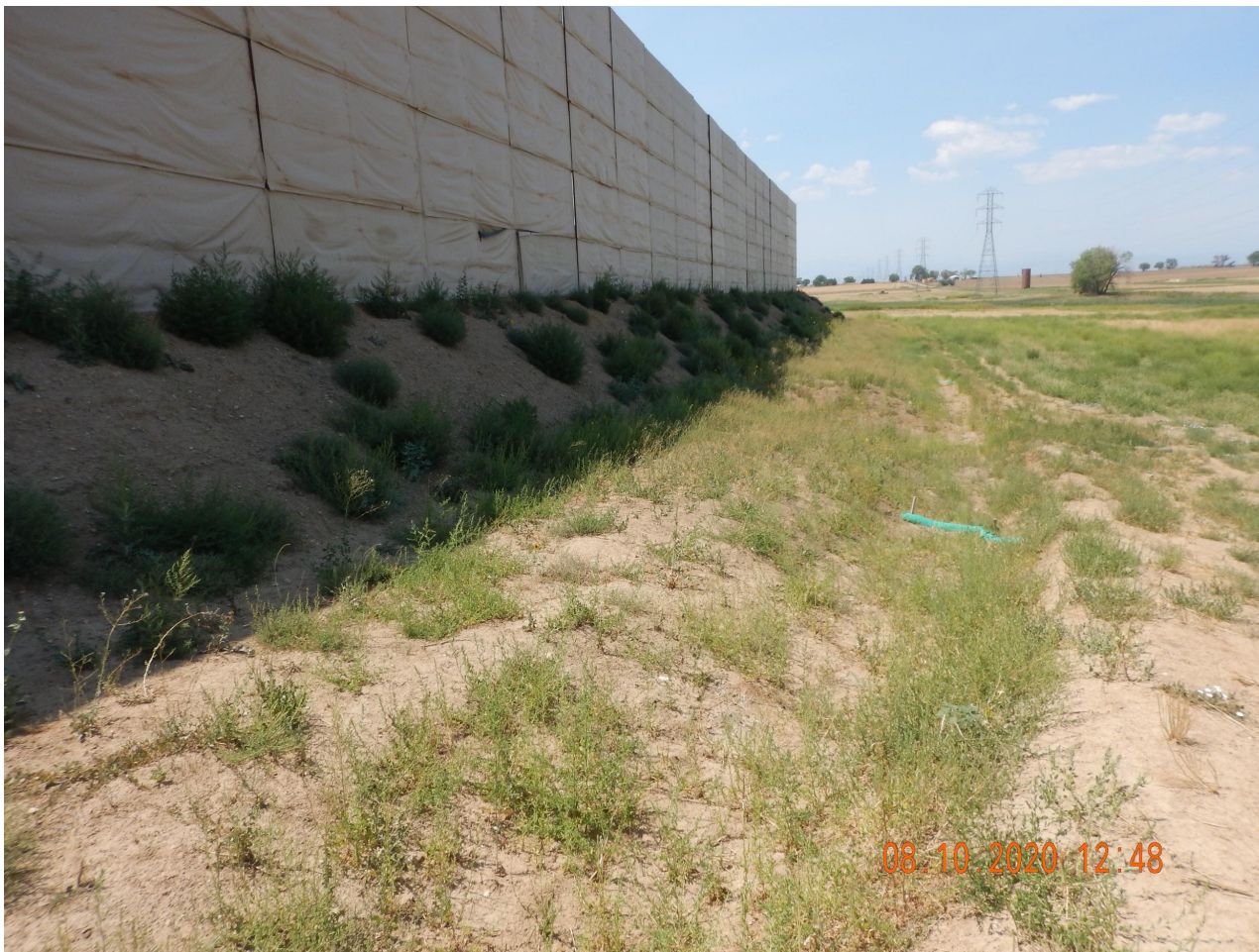
Photo 4. Photo taken from the northeastern location, facing West. Photo illustrates the Operator has repaired erosion along the northern fill slope.
