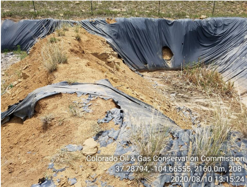
PHOTO 3: PIT LINER IS IN DISREPAIR. REMOVE OR REPLACE LINER, COMPLY WITH RULE 904. CA DATE 11-11-20.
