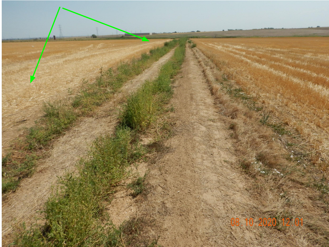
Photo 1. Photo taken from the western access road, facing East. Photo illustrates the Operator has failed to recontour the access road, as well as control undesirable weeds. Note- it does not appear the surface owner is using the access road; surface owner is driving north of the access road with the evidence of agricultural activities (green arrows). Also, refer to Photos 4-6.
