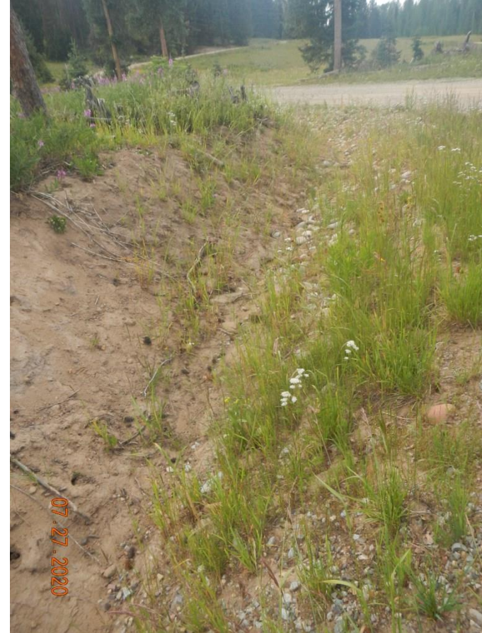
Photo#5: Amount of sediment migration is occurring along access road ditches and base of cut.
