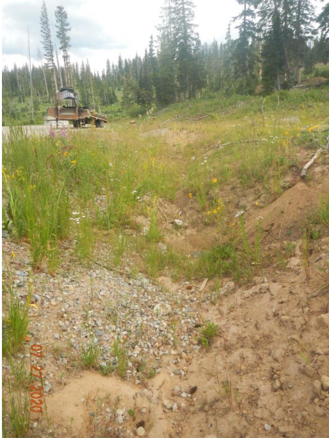
Photo#4: Amount of sediment migration is occurring along access road ditches and base of cut.
