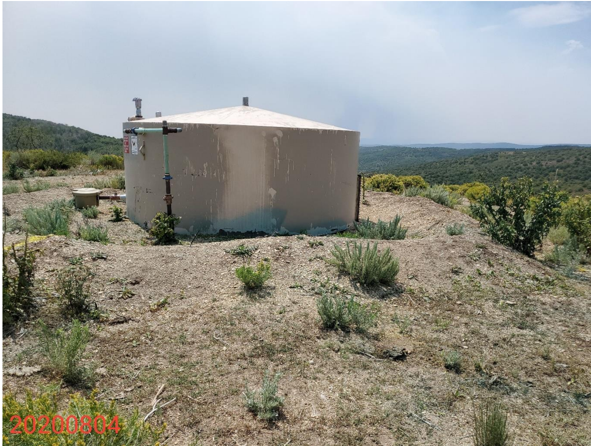
Photo 3: Photo of 200 bbl condensate tank. Photo shows vegetative establishment within and on secondary containment. Vegetative establishment within compromises the imperviability of the containment per rule 906.d.(1). Containment BMP does not appear to be sufficient to contain contents of tank and sufficient freeboard to contain precipitation.
