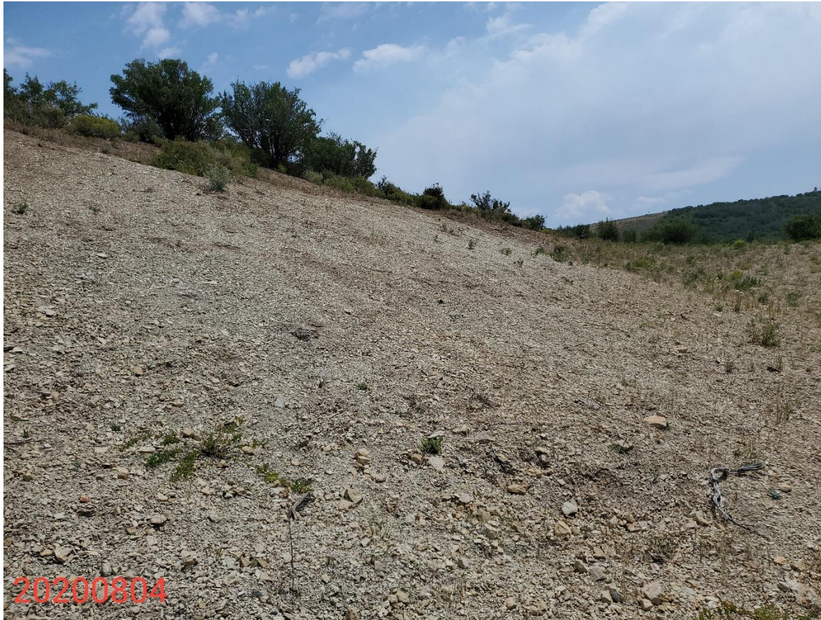
Photo 9: Photo taken from the wester interim areas. Photo shows BMPs missing or insufficient to stabilize soils on slope. Photo also shows interim areas are not progressing towards 1003 standards.
