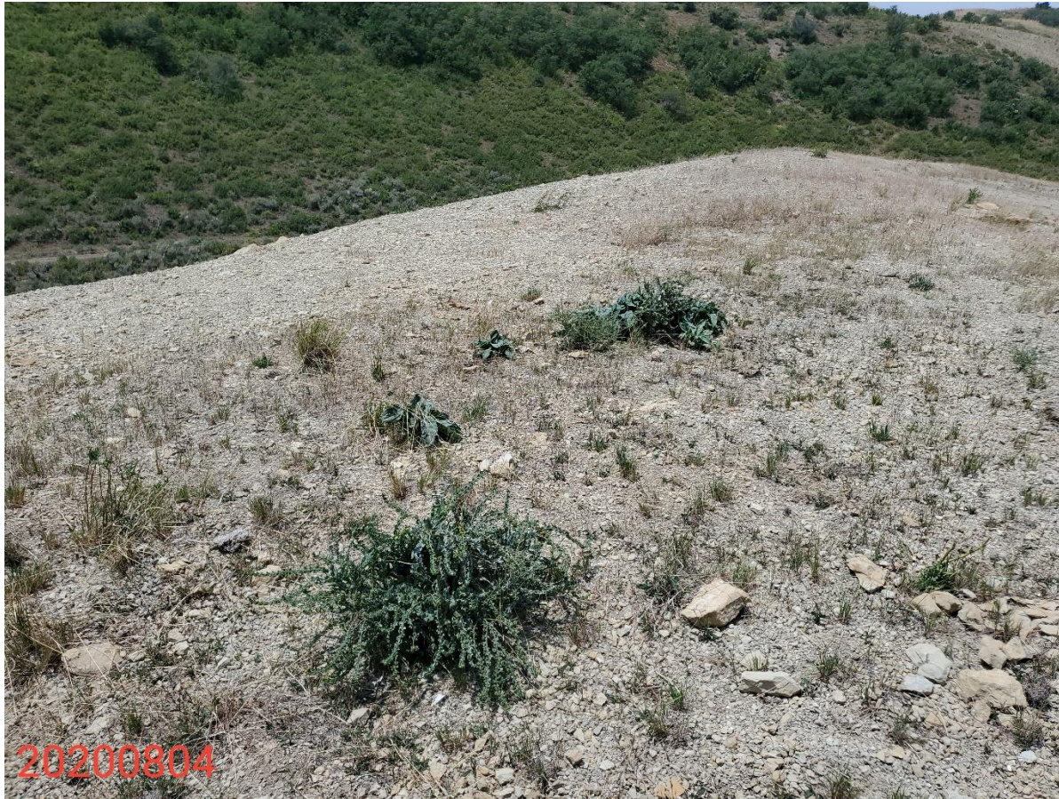
Photo 10: Photo taken the interim areas on the south end of the Location, facing southwest. Photo shows BMPs missing or insufficient to stabilize soils on slope. Photo also shows interim areas are not progressing towards 1003 standards, and noxious weeds.
