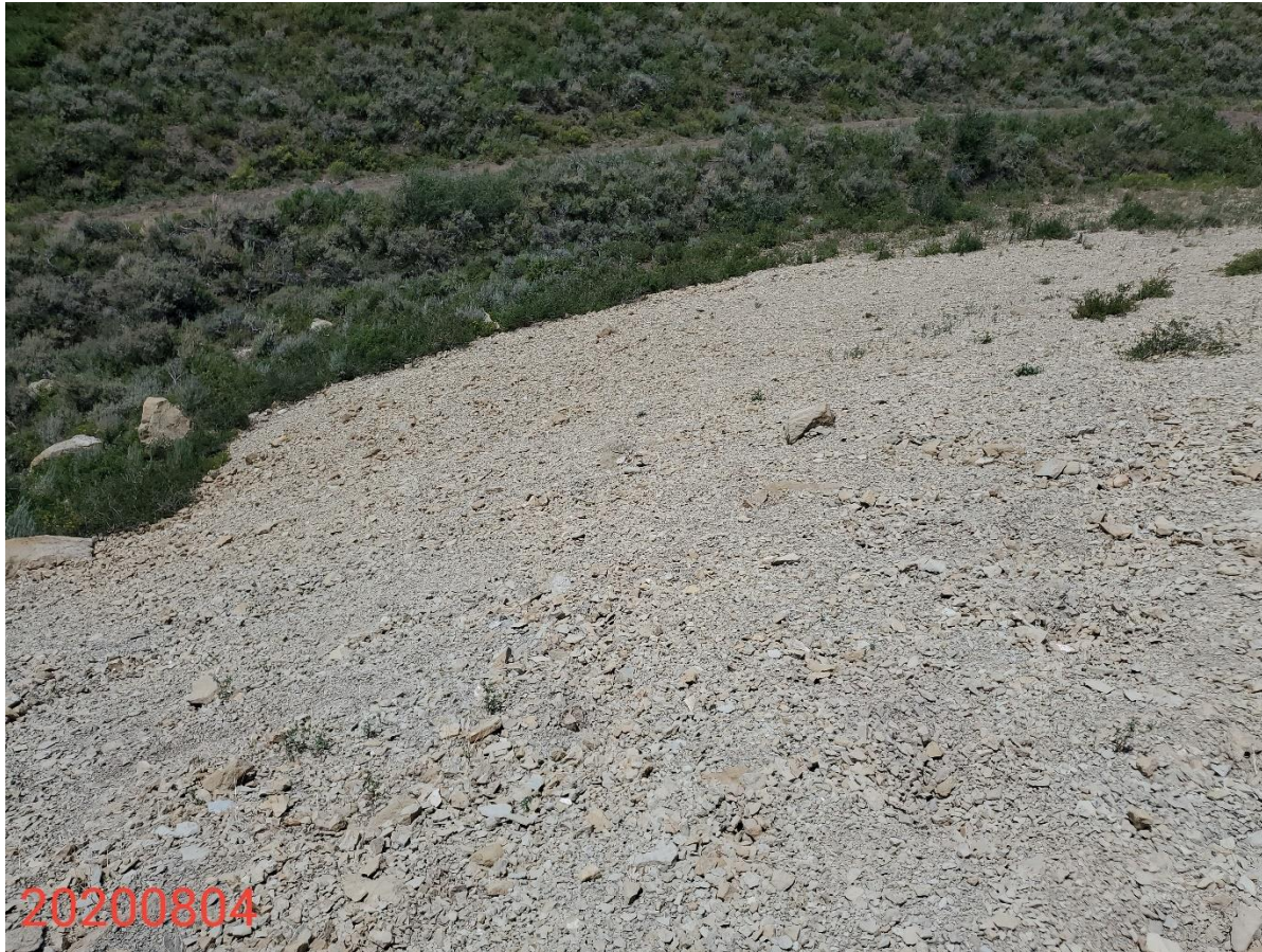
Photo 12: Photo taken the interim areas on the west end of the Location, facing west. Photo shows BMPs missing or insufficient to stabilize soils on slope. Photo also shows interim areas are not progressing towards 1003 standards.
