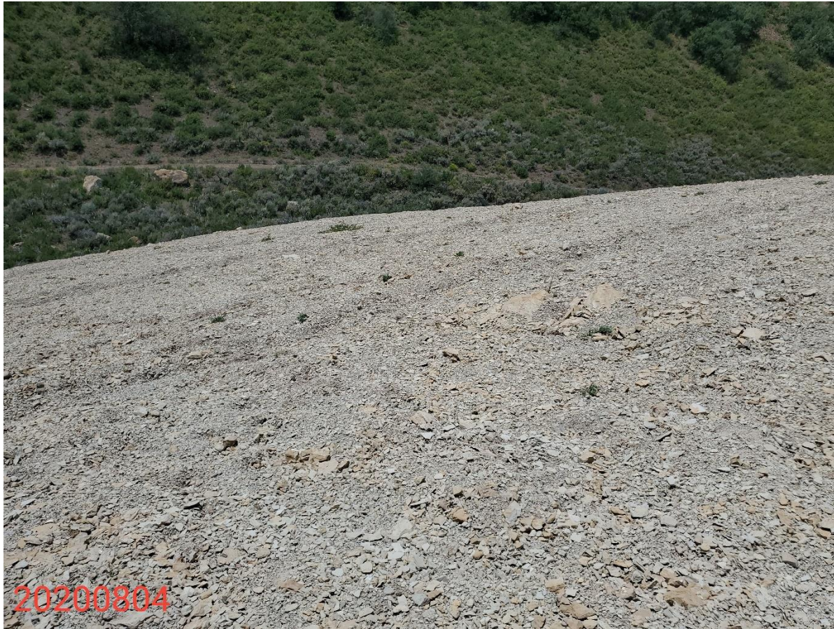
Photo 11: Photo taken the interim areas on the south end of the Location, facing southwest. Photo shows BMPs missing or insufficient to stabilize soils on slope. Photo also shows interim areas are not progressing towards 1003 standards.
