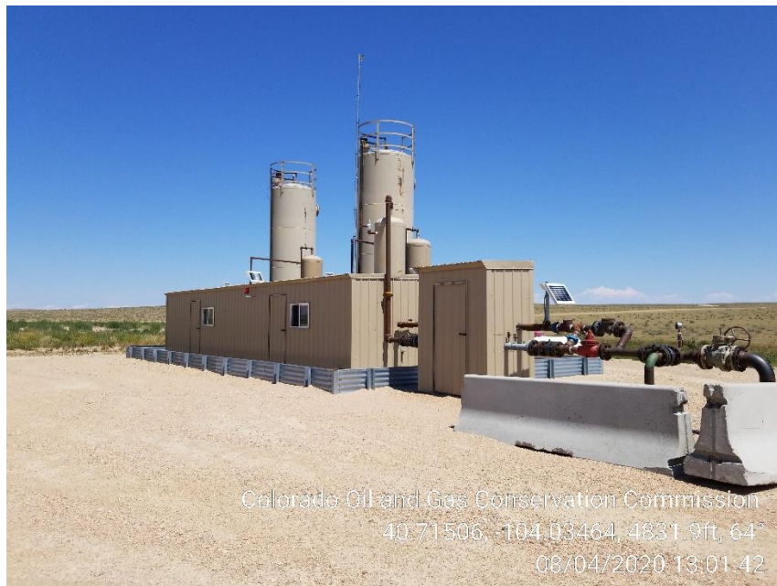
Photo 5 – East Heater Treaters
