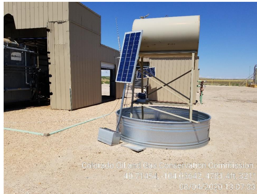
Photo 8 – Methanol Missing Wildlife Netting
