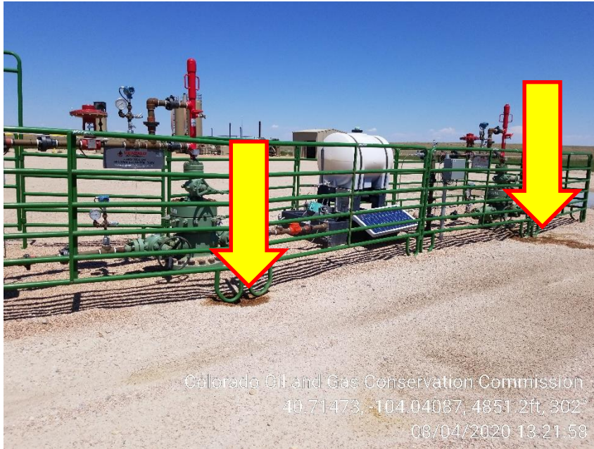
Photo 1 – Wellheads, Stained Soil
