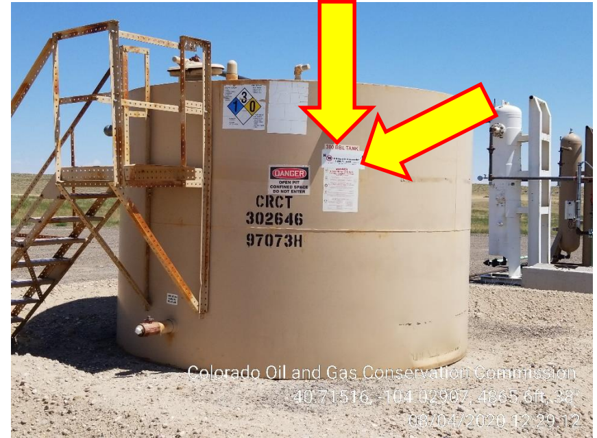
Photo 2 – Maintenance Tank, Current 24 Hour Emergency # missing, Capacity not current, Content missing
