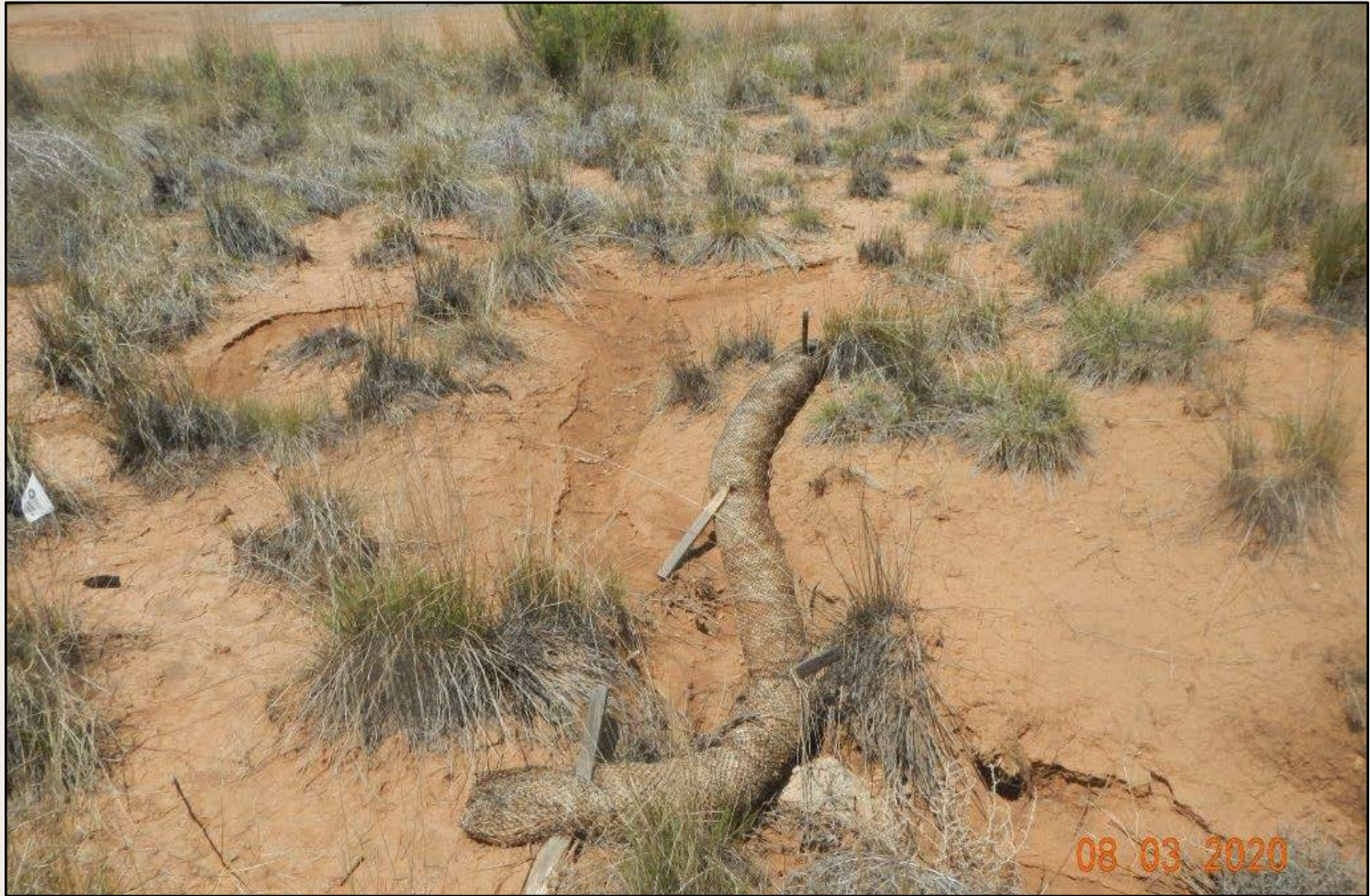
Photo 3. View of wattles that are no longer functioning within the eastern project area.
