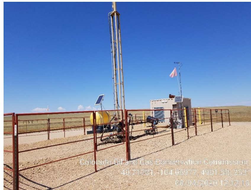
Photo 2 – Hydraulic Pumping Unit
