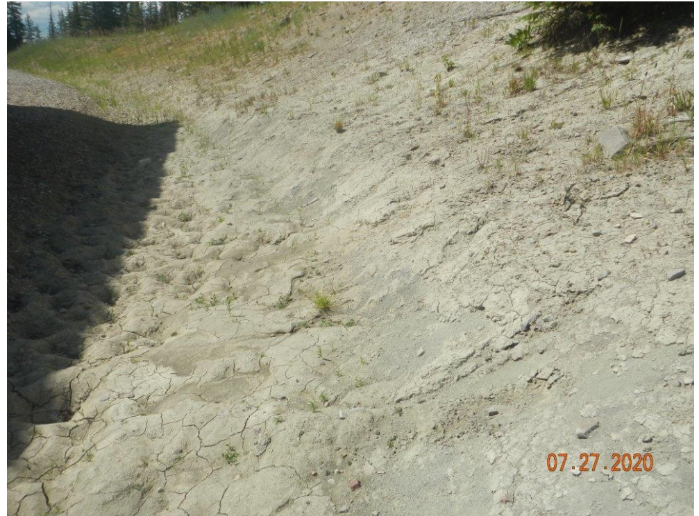
Photo#5: Initiation of erosion on Cut slope.
