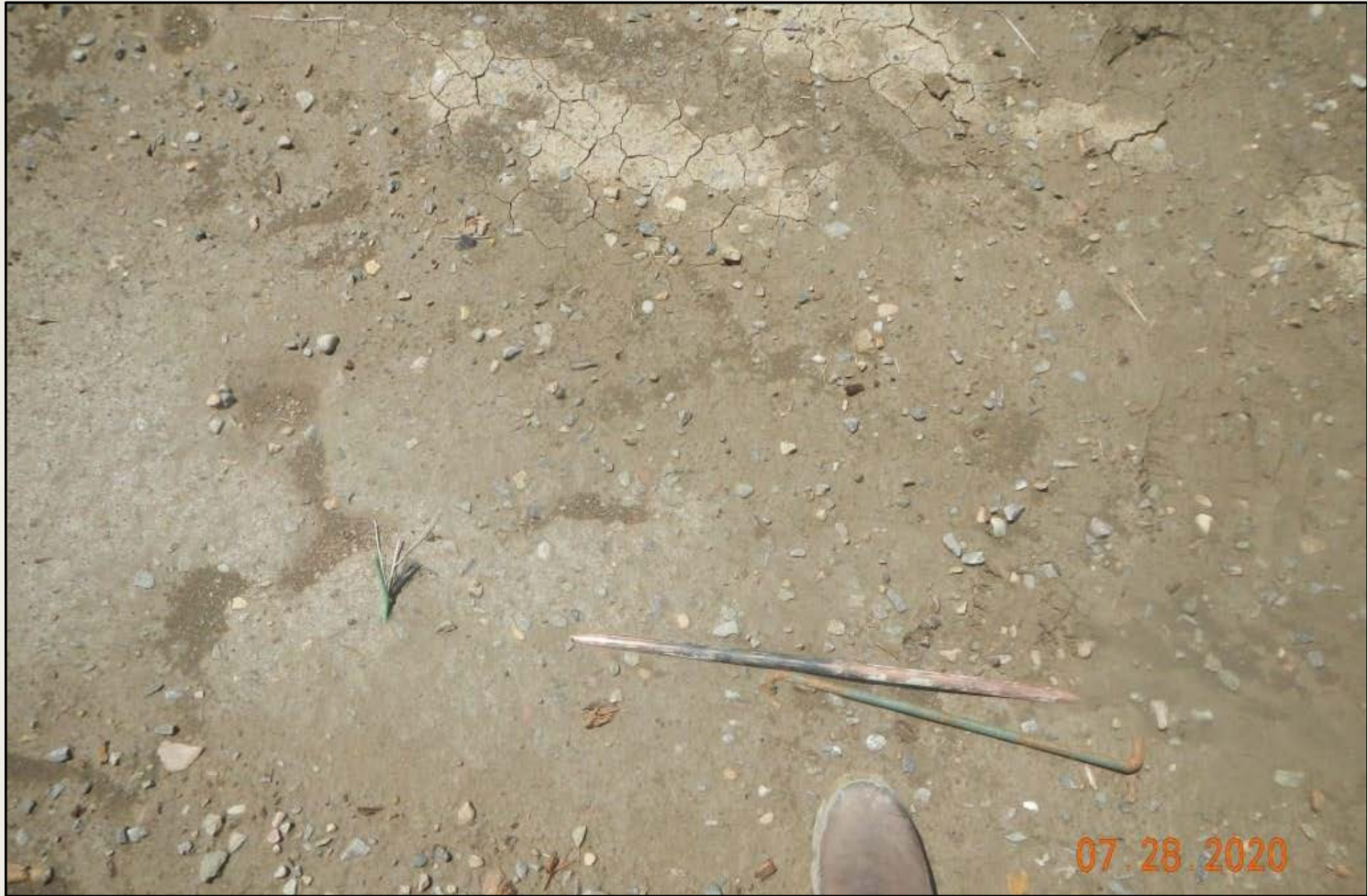
Photo 2. View of exposed pipe and wiring on the well pad, needing to be removed.
