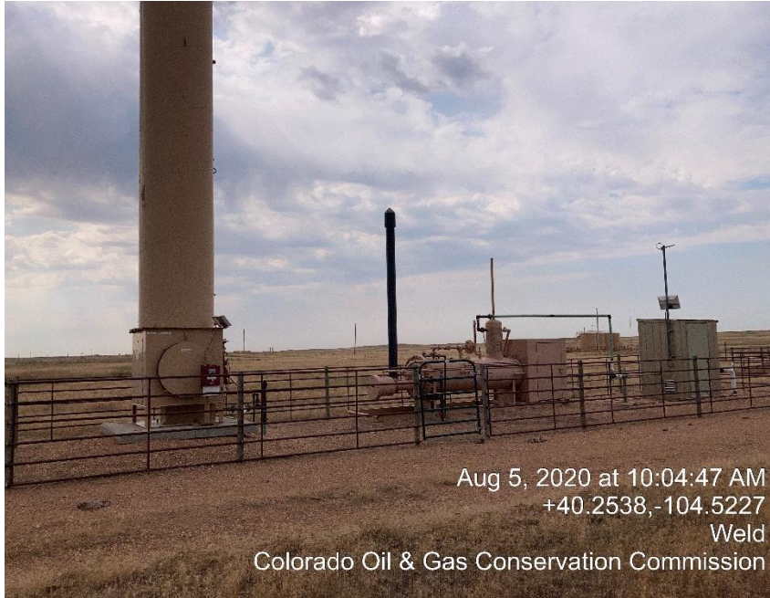
Photo #3 Separator, ECD & Meter Run
